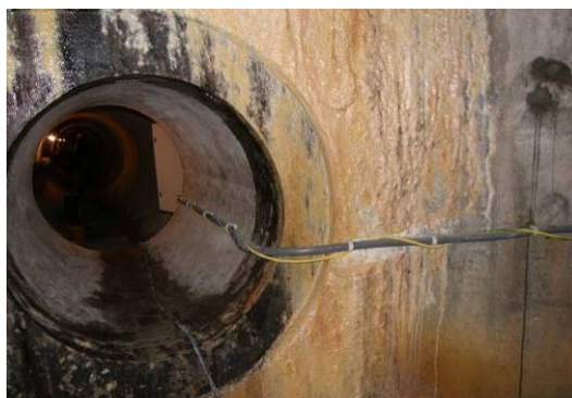
Figure 35. The conduit containing the anode header cable, cathode header cable, and rebar cable. The unit is powered by the yellow extension cord wrapped around the conduit.
