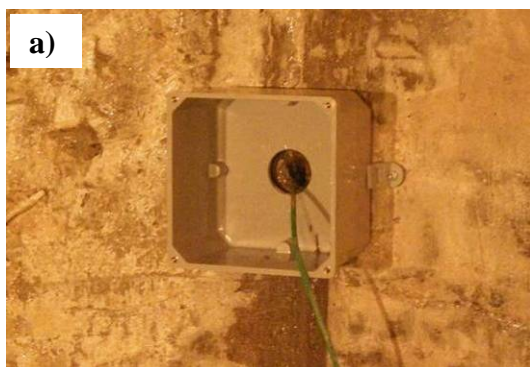
Figure 29. Installation of junction boxes and wiring of system.
