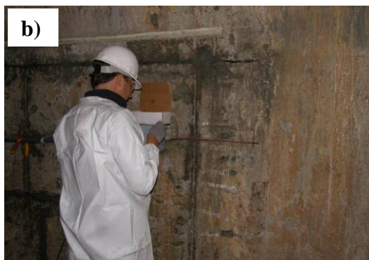
Figure 31. Anode cables were embedded into the wall to the cathode junction box, and cable was run through the same conduit as the cathode cables.
