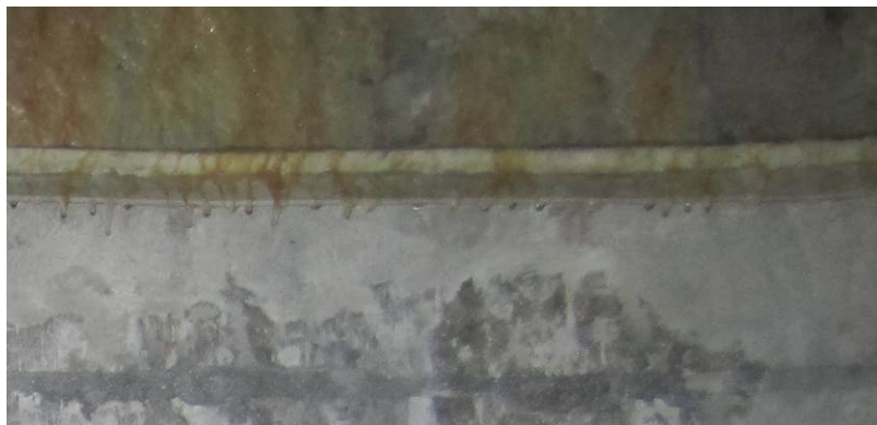
Figure 44. Visible water overflowing the drip tray, allowing water to fall onto the wall and junction boxes below. Note the color of the streaks of water, indicating that the water is rich in calcium carbonate.
