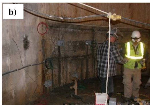
Figure 30. Cables were run through conduit to main junction box.
