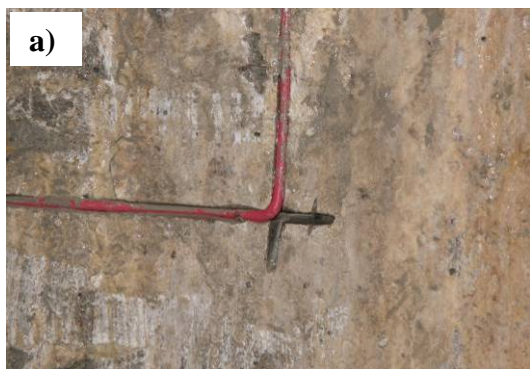
Figure 31. Anode cables were embedded into the wall to the cathode junction box, and cable was run through the same conduit as the cathode cables.
