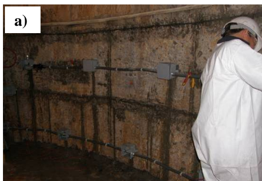
Figure 30. Cables were run through conduit to main junction box.
