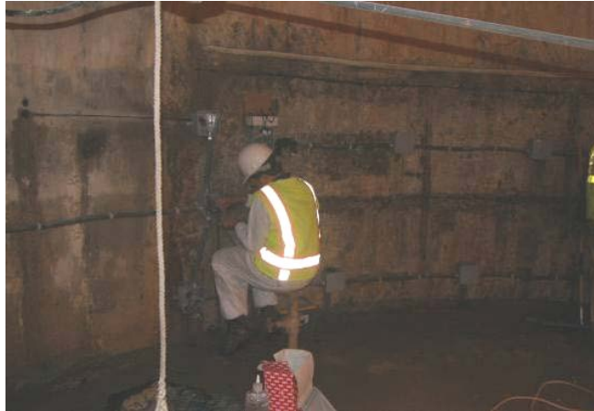
Figure 32. All cables were terminated in a main junction box. The cathode cables were connected to a main cathode header cable, all the anode cables were connected to a main anode header cable, and the main header cables and a cable connected to the rebar were run through conduit to the system controller.
