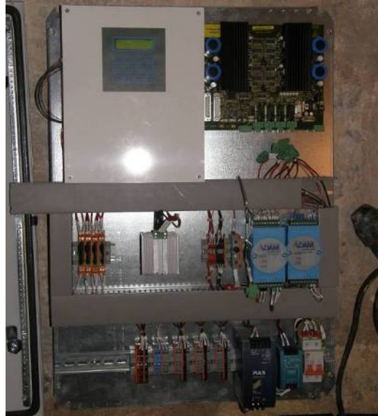
Figure 17. DC voltage controlled pulse unit installed at Trinity Dam for the EOP system.
