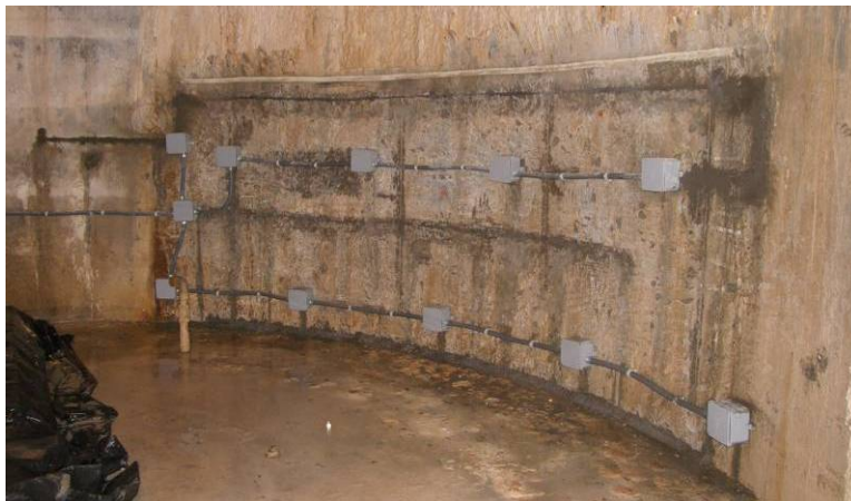
Figure 33. Completed installation with junction boxes and conduit.
