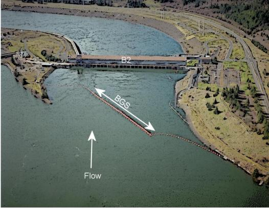
Figure 2. The Behavioral Guidance Structure (BGS) with One Section Shown out of the Water (above); and Shown Deployed in the Forebay of the Bonneville Dam Second Powerhouse (B2; below).
