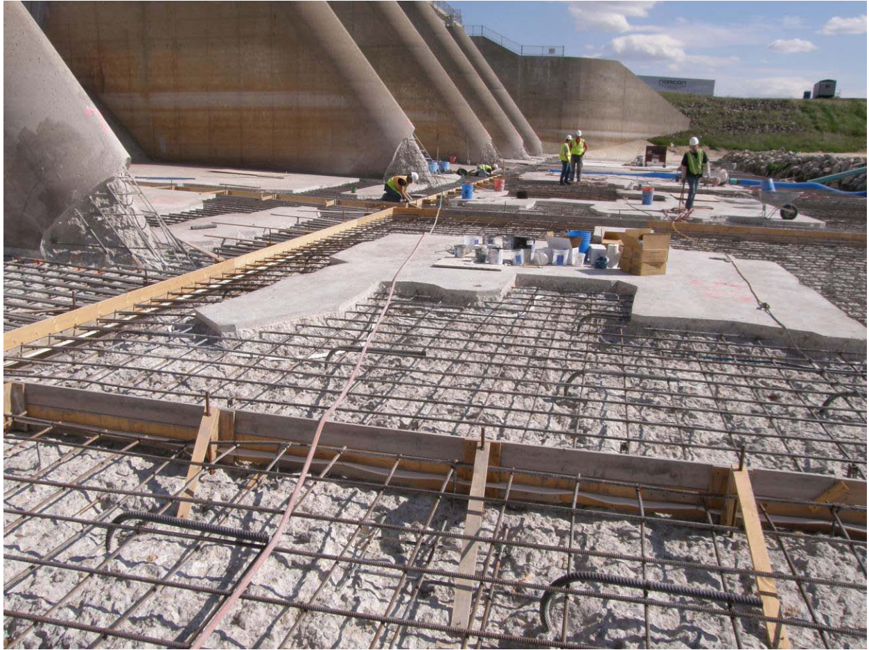
Figure 6. – Example of concrete removal with some original concrete remaining.
