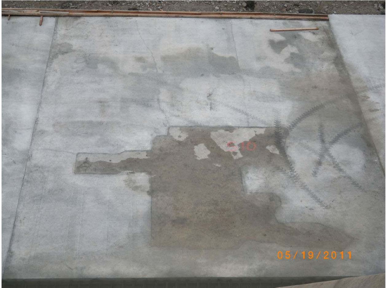
Figure 17. – Slab 10 repair made with the trial concrete.
