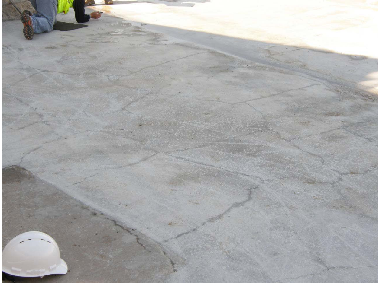
Figure 13. – Typical shrinkage cracking that was measured and mapped.
