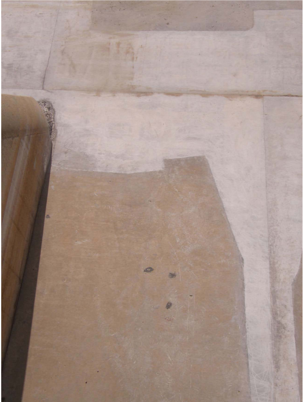
Figure 11. – Bay 7 placement made with concrete without the Premier Magnesia additive.
