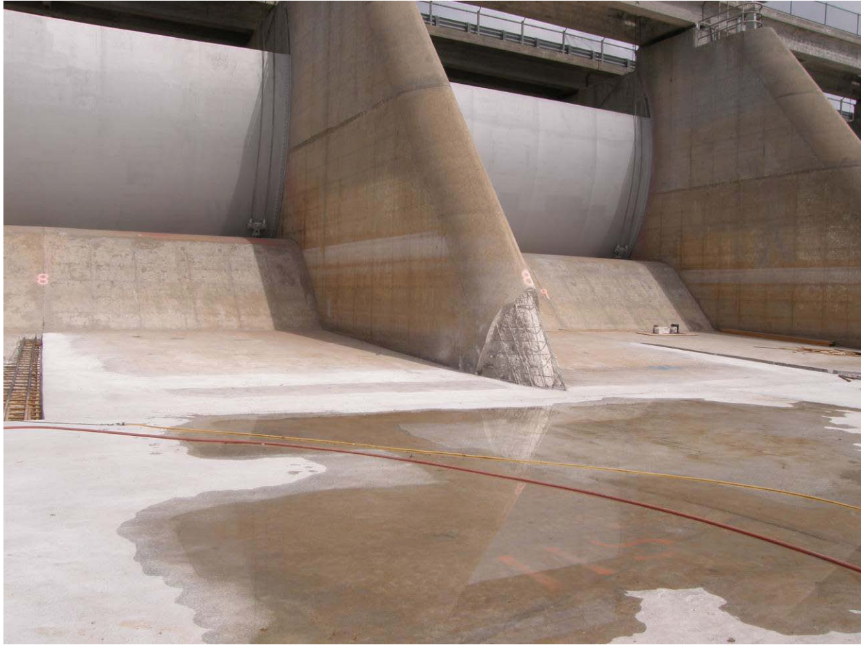
Figure 12. – Placement B8/9 made with concrete containing the Premier Magnesia additive.
