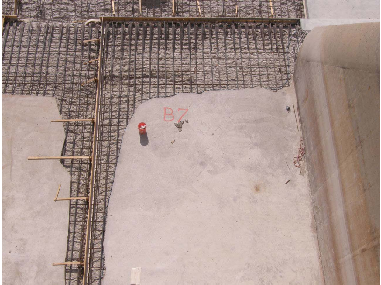
Figure 8. Bay 7 ready for trial concrete placement using concrete containing the Premier Magnesia additive.
