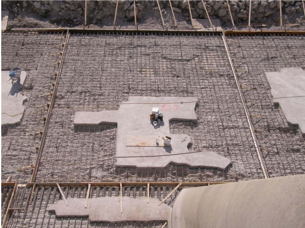
Figure 9. – Slab 10 ready for trial concrete placement using concrete containing the Premier Magnesia additive.
