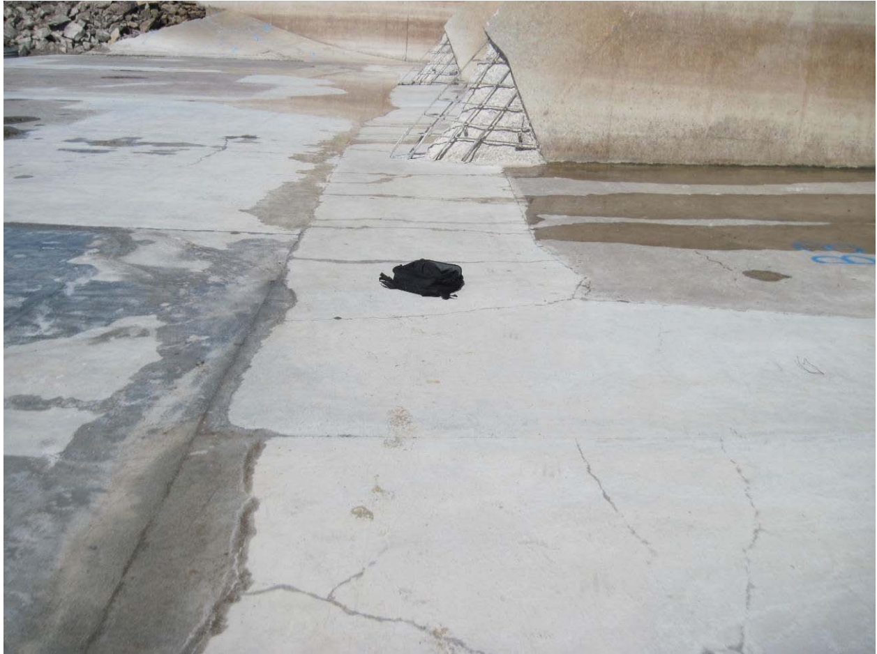
Figure 7. – View of shrinkage cracking first observed within one to two weeks of concrete placement.
