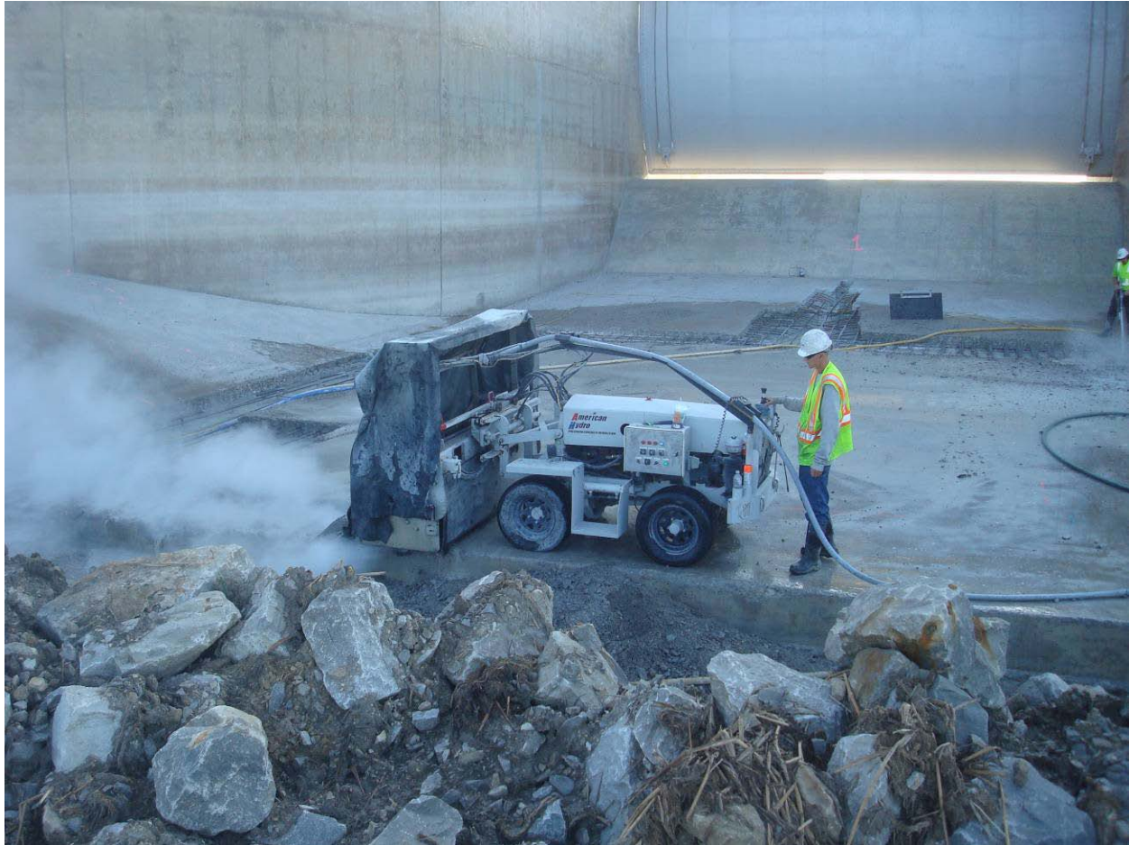
Figure 5. – Hydrodemolition of damaged concrete
