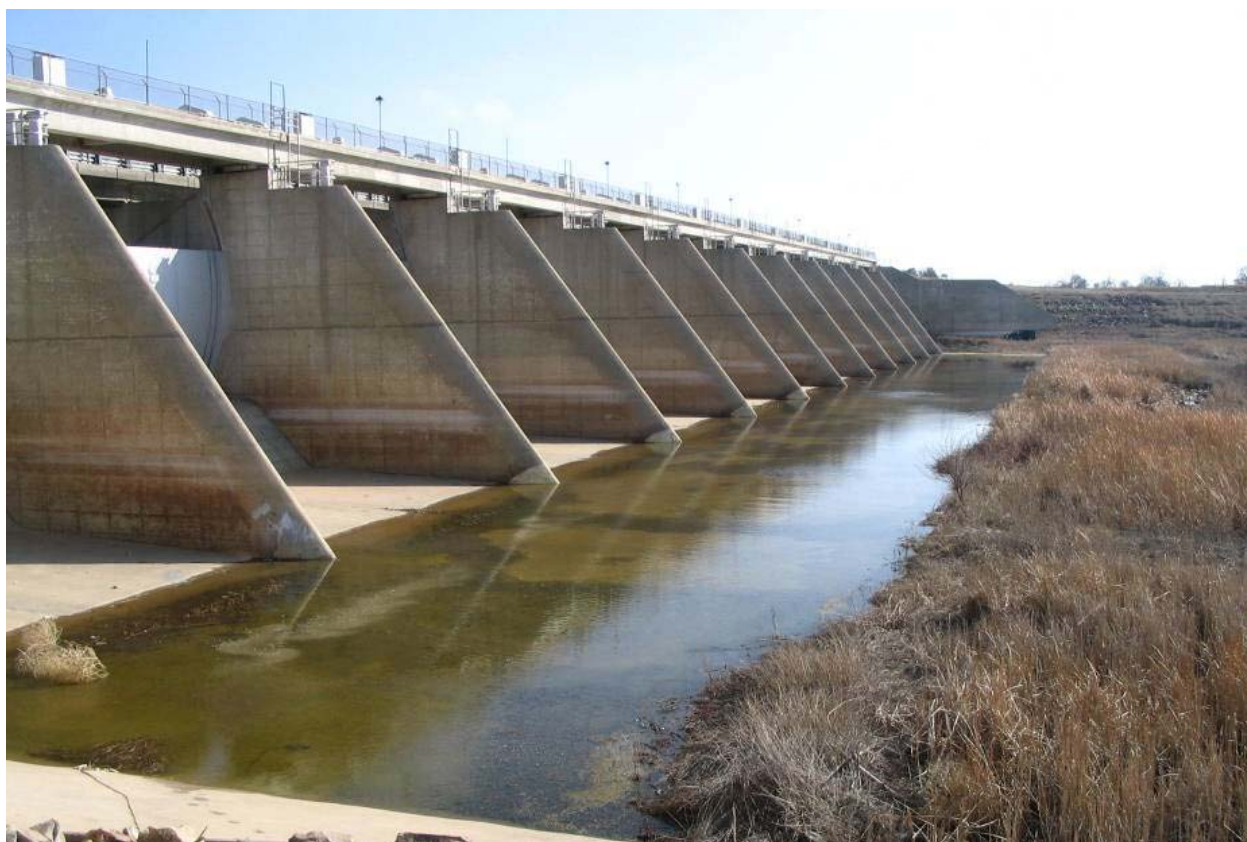
Figure 2. – View of approach area of spillway. The soil berm trapped water on the apron, leading to deterioration of the concrete.
