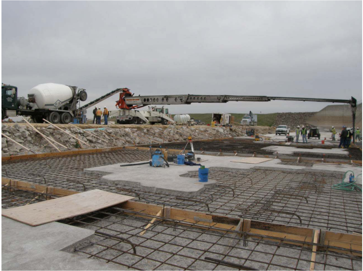
Figure 16. – Placement of the trial concrete.
