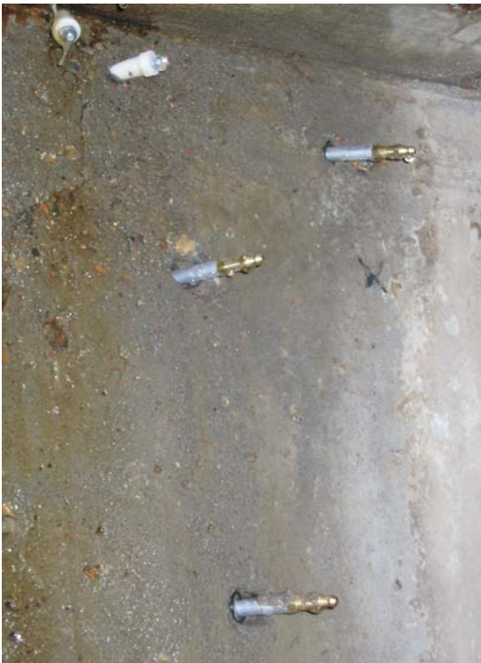
Figure 10. - In several locations, combinations of bang-in and mechanical packers were used to assist with grout injection.
