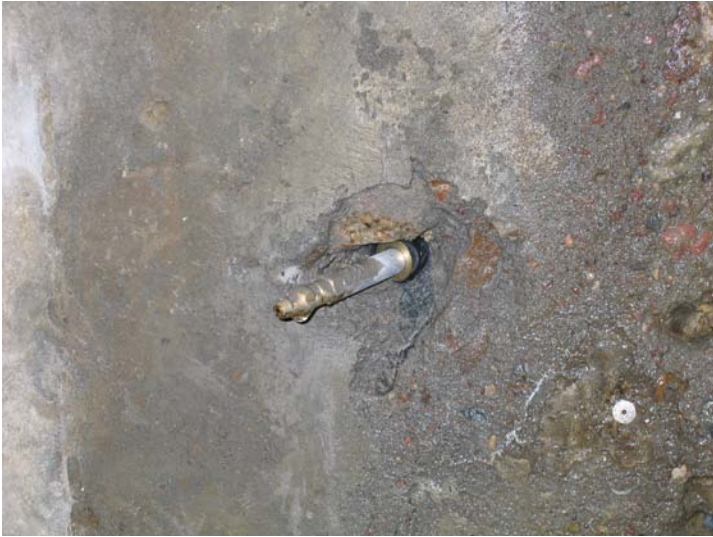
Figure 7. - A mechanical packer with a longer tube, useful for insertion into deeper holes. Note water dripping from end, indicating water bearing crack has been intercepted.
