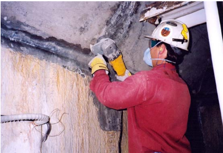
Figure 8. - Grinding surface deposits from face of crack.
