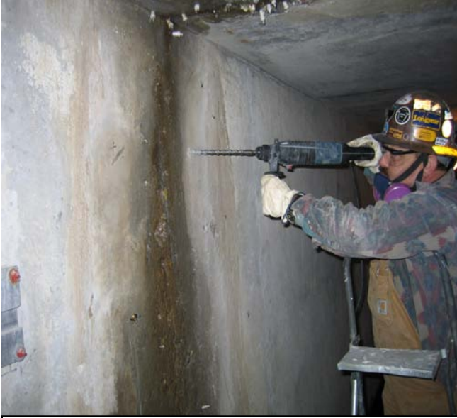
Figure 9. - Drilling holes for mechanical packers.
