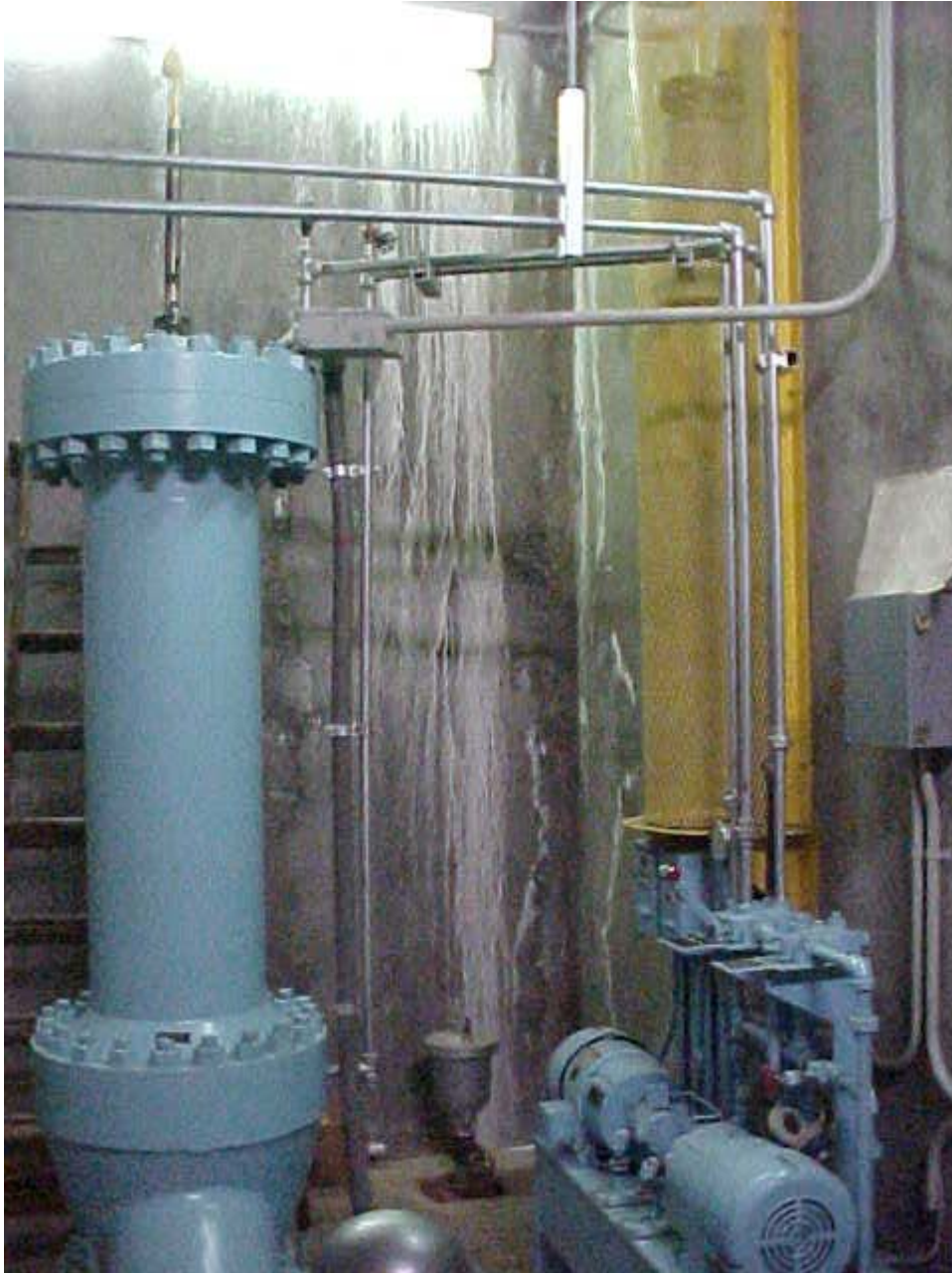
Figure 9. - Buttress 16 gate and equipment gallery water leaks.
