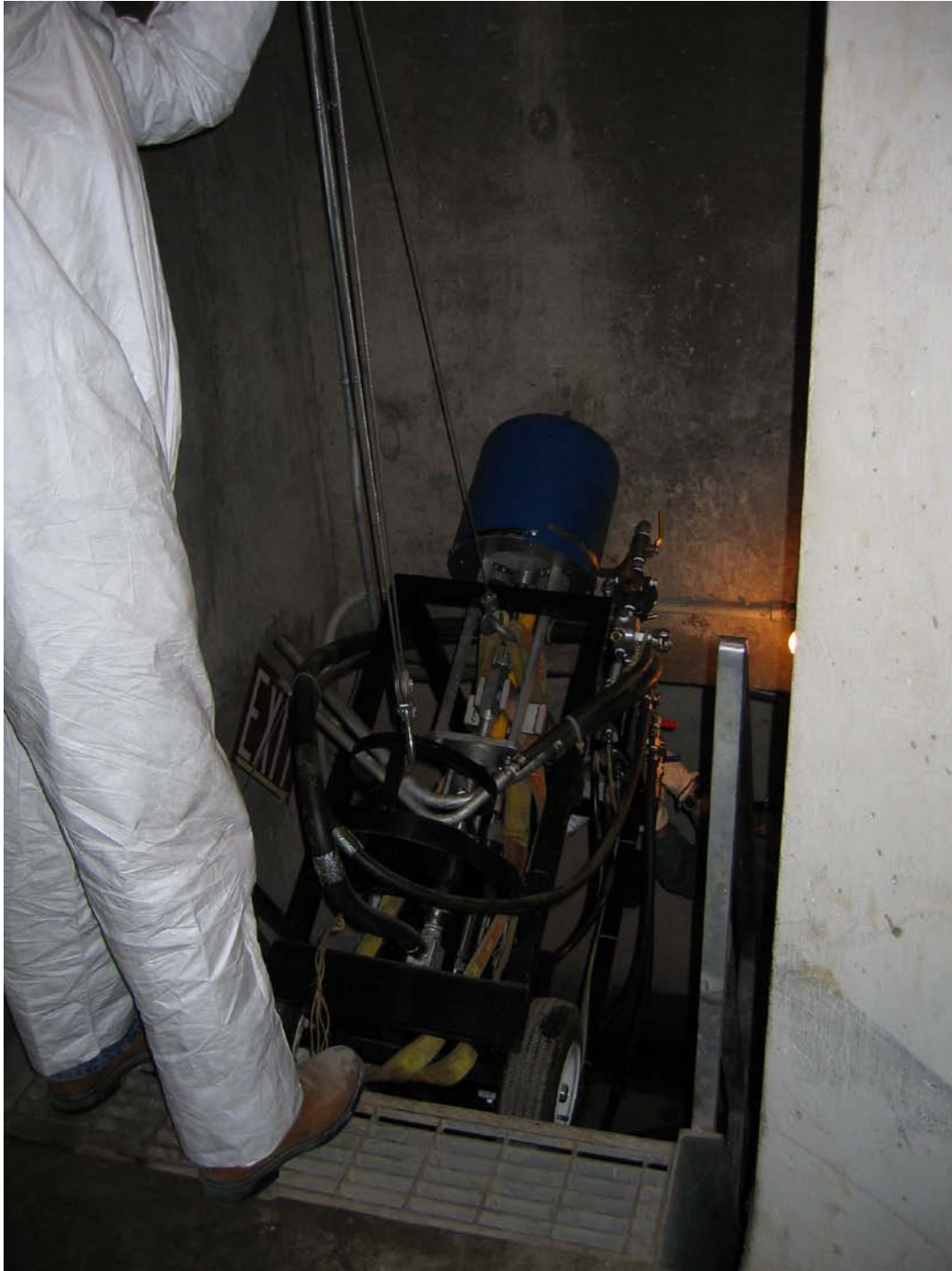
Figure 14. - Lowering the rocker pump into a gallery.
