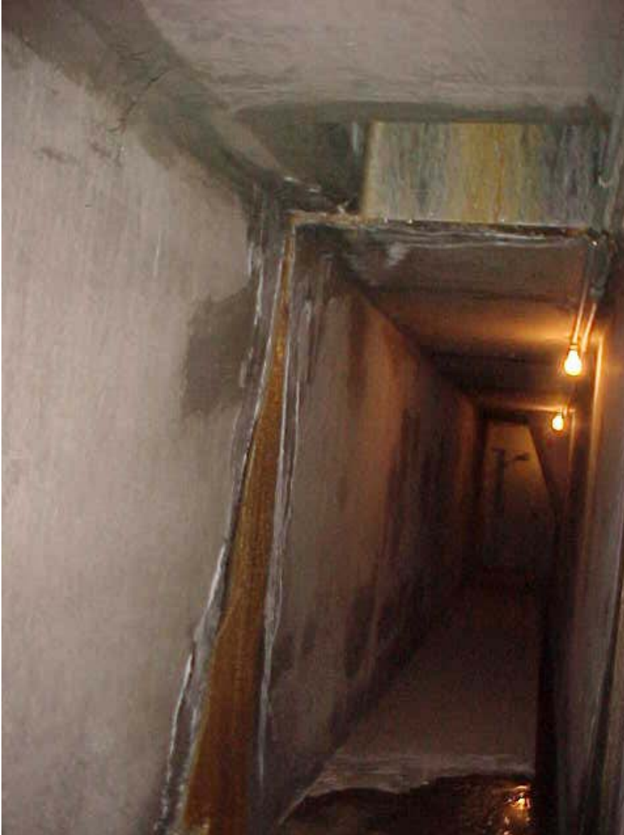
Figure 5. - Buttress 8 equipment area water leaks.
