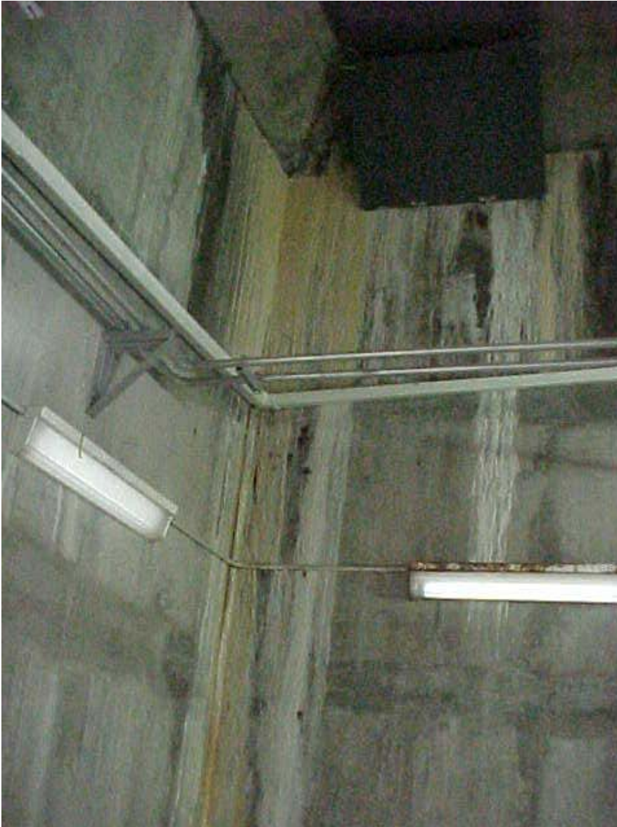
Figure 7. -Buttress 11 gate chamber water leaks through joints.
