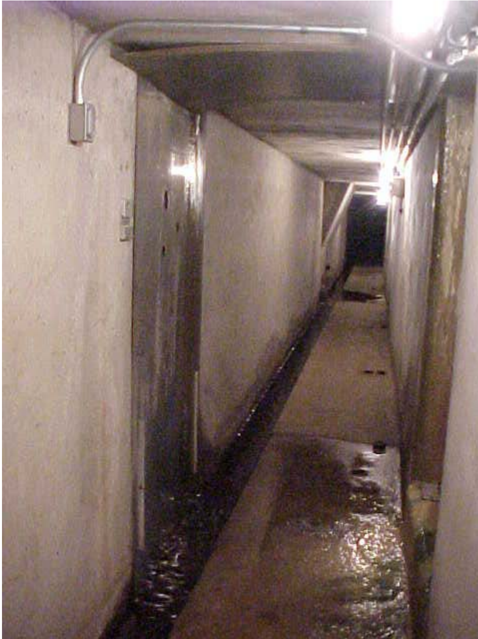
Figure 7. -Buttress 10 inspection and equipment gallery area water leaks.
