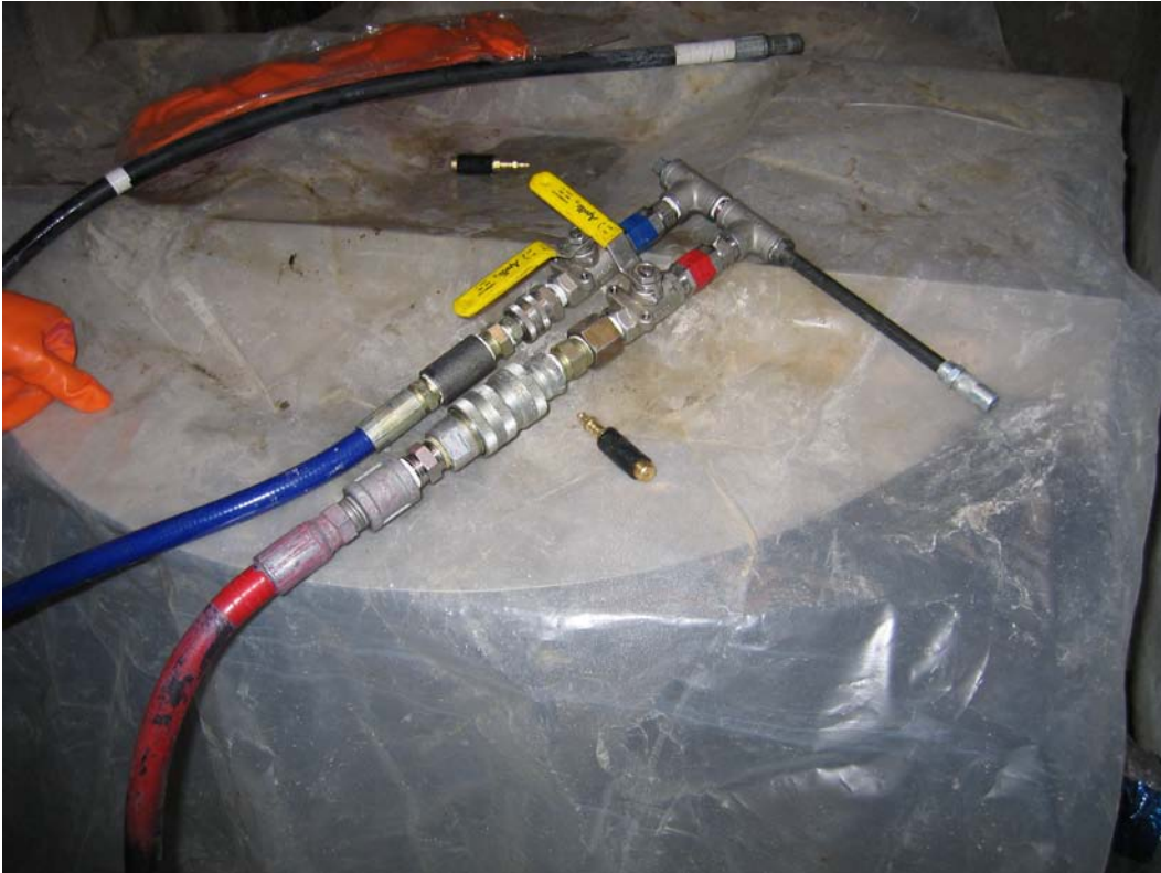
Figure 12. - Assembly used to connect grout lines to injection ports for higher pressure injection. Note provision for 2 material lines, which allows for keeping reacting materials separate until close to the point of injection. A small chain or mixer in the small tube provides for mixing just prior to injection.
