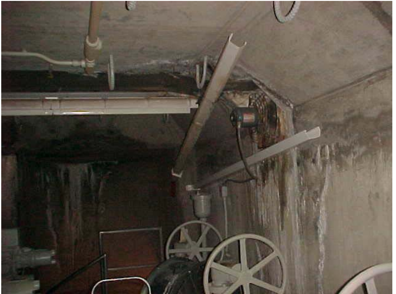
Figure 4. - Fish hatchery outlet works gate chambers water leaks.
