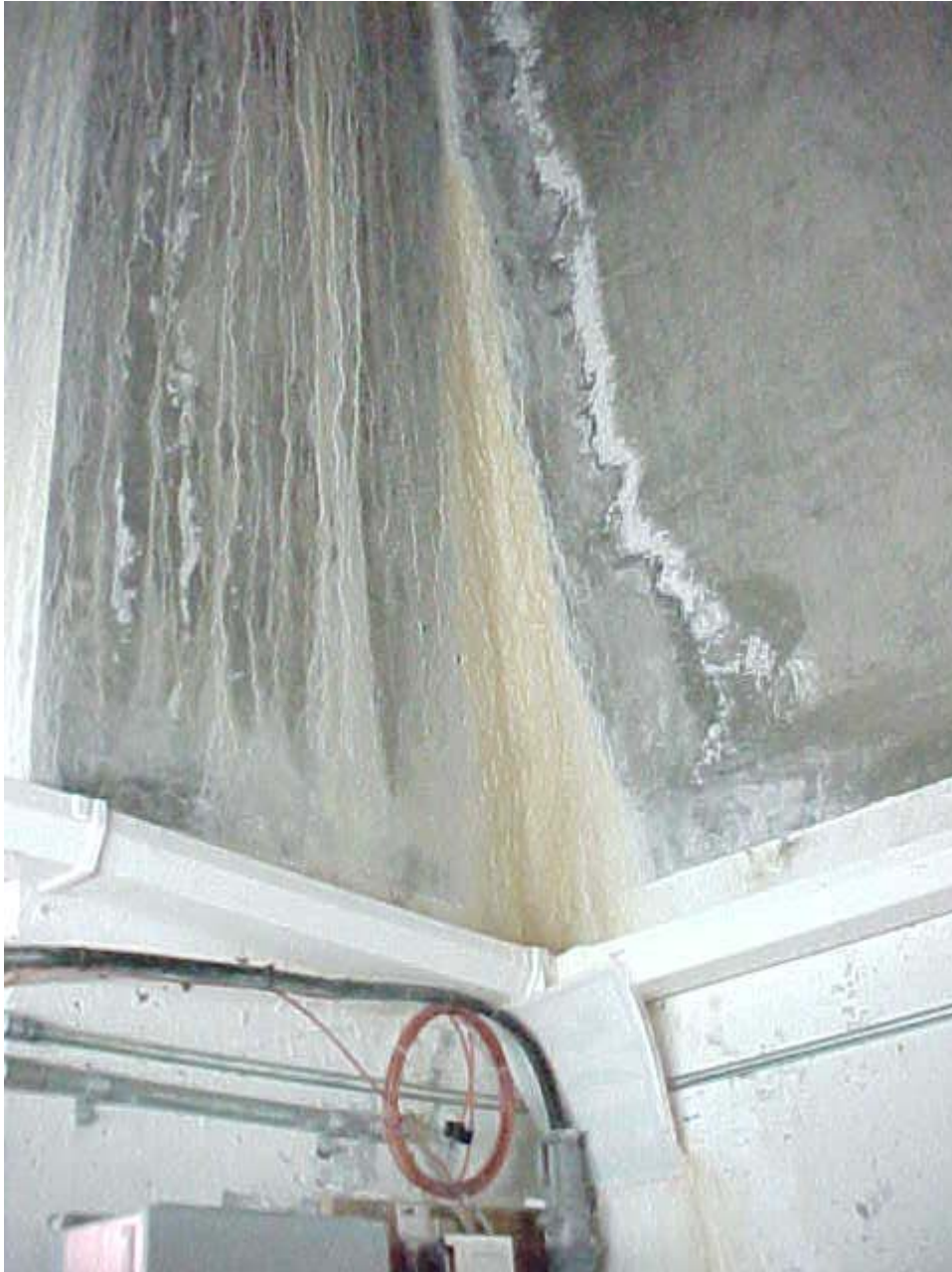
Figure 6. - Buttress 17 entry adit water leaks.
