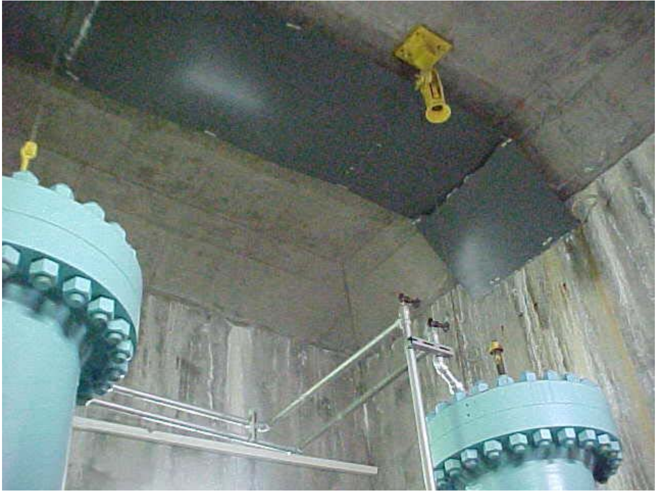
Figure 8. - Buttress 13 gate chamber leak and water deflection sheeting across roof.
