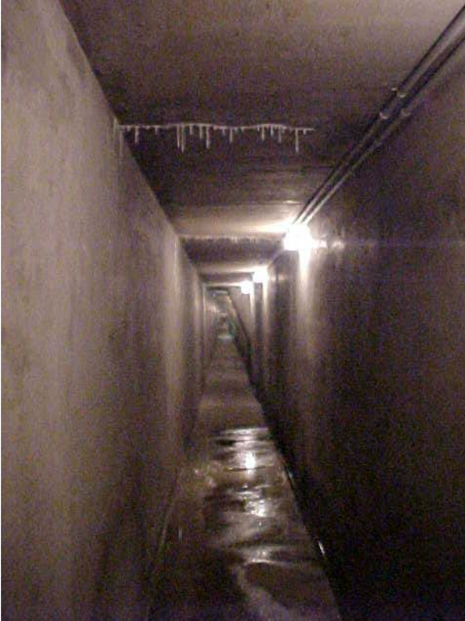
Figure 8. Buttress 15 inspection and equipment gallery area water leaks.
