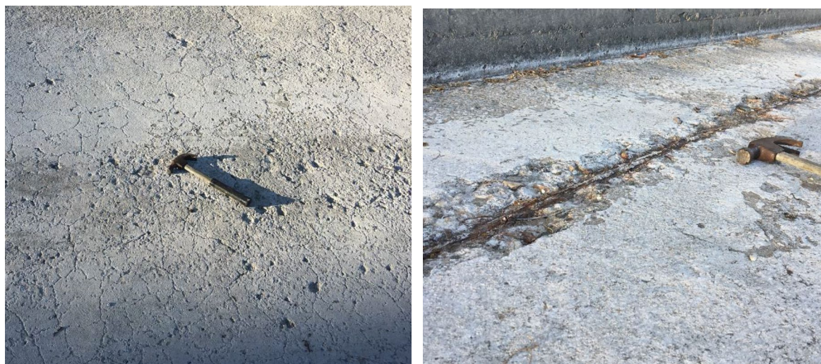
Figure 4. Typical cracking and deterioration along spillway chute at Bradbury Dam.
