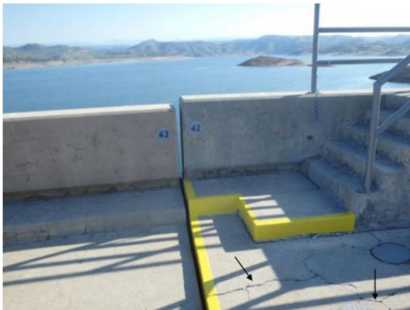
Figure 3. Concrete at Friant Dam with pumicite (left) and without pumicite (right). Arrows pointing to map cracking indicative of ASR.
