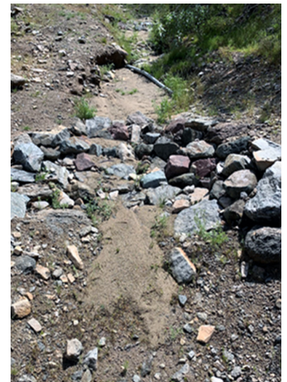
Grade Control Structure #1 looking upstream, March 13, 2020. (Bureau of Reclamation photo, Phoenix Area Office, Deborah Tosline)
