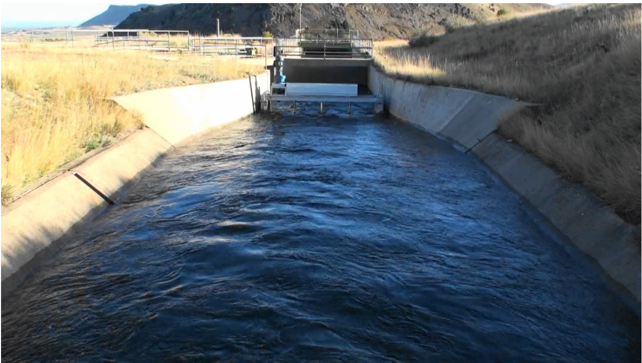
Figure 34 HK #4 (Zone B station 0) operating at 266 ft 3 /s, looking downstream.
