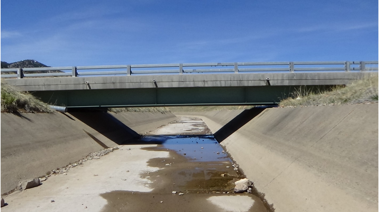
Figure 33 Zone B canal with trapezoidal cross section. At station 64, looking upstream.
