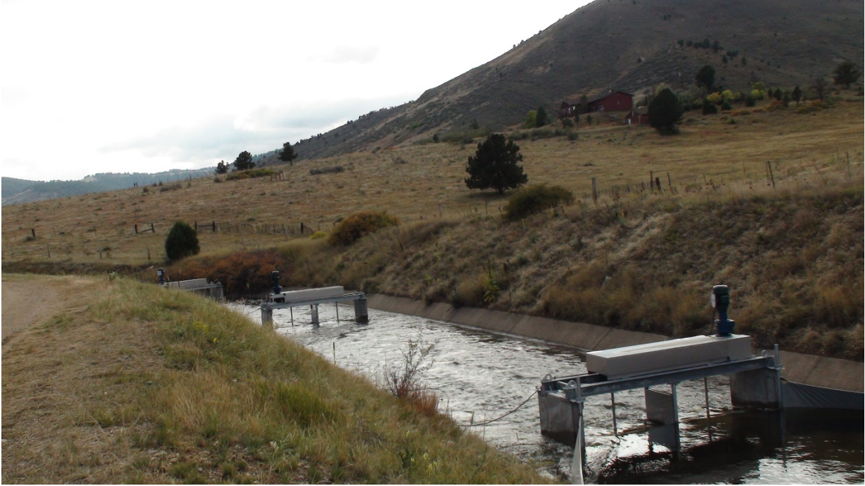
Figure 37 HK #'s 7, 8, and 9 (Zone B stations 750, 823, and 890 ft, respectively) operating at 266 ft 3 /s, looking downstream.
