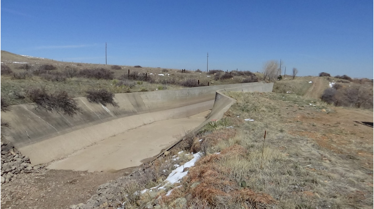
Figure 41 Rectangular Bench flume that crosses a ravine in Zone C (station 4,000 ft), looking upstream.
