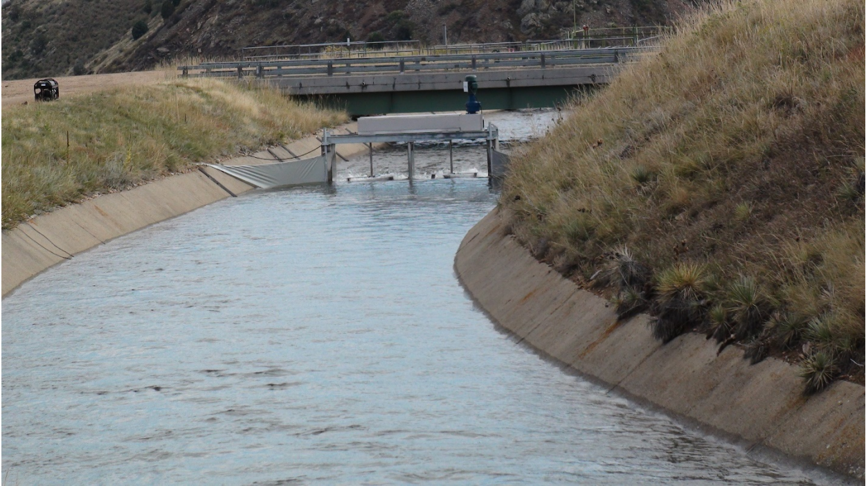
Figure 35 HK #5 (Zone B station 250 ft) operating at 266 ft 3 /s, looking downstream.
