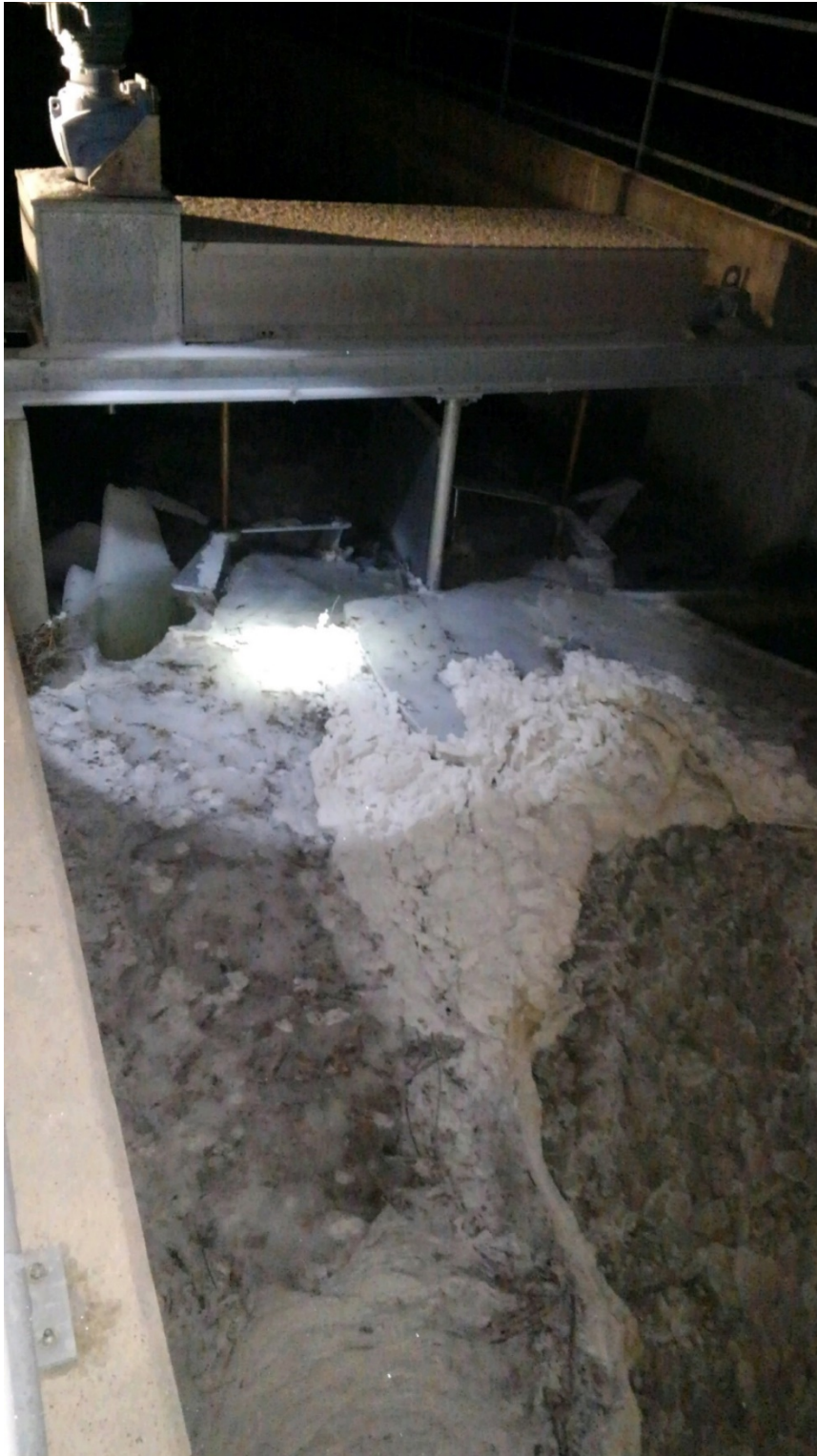
Figure 24 Ice upstream of an HK unit in Zone A, looking downstream.
