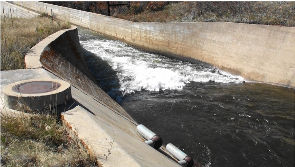
Figure 42 Supercritical flow and hydraulic jump entering Zone C bench flume at 266 \text{ ft}^3/\text{s} (station 4,300 ft), looking downstream.
