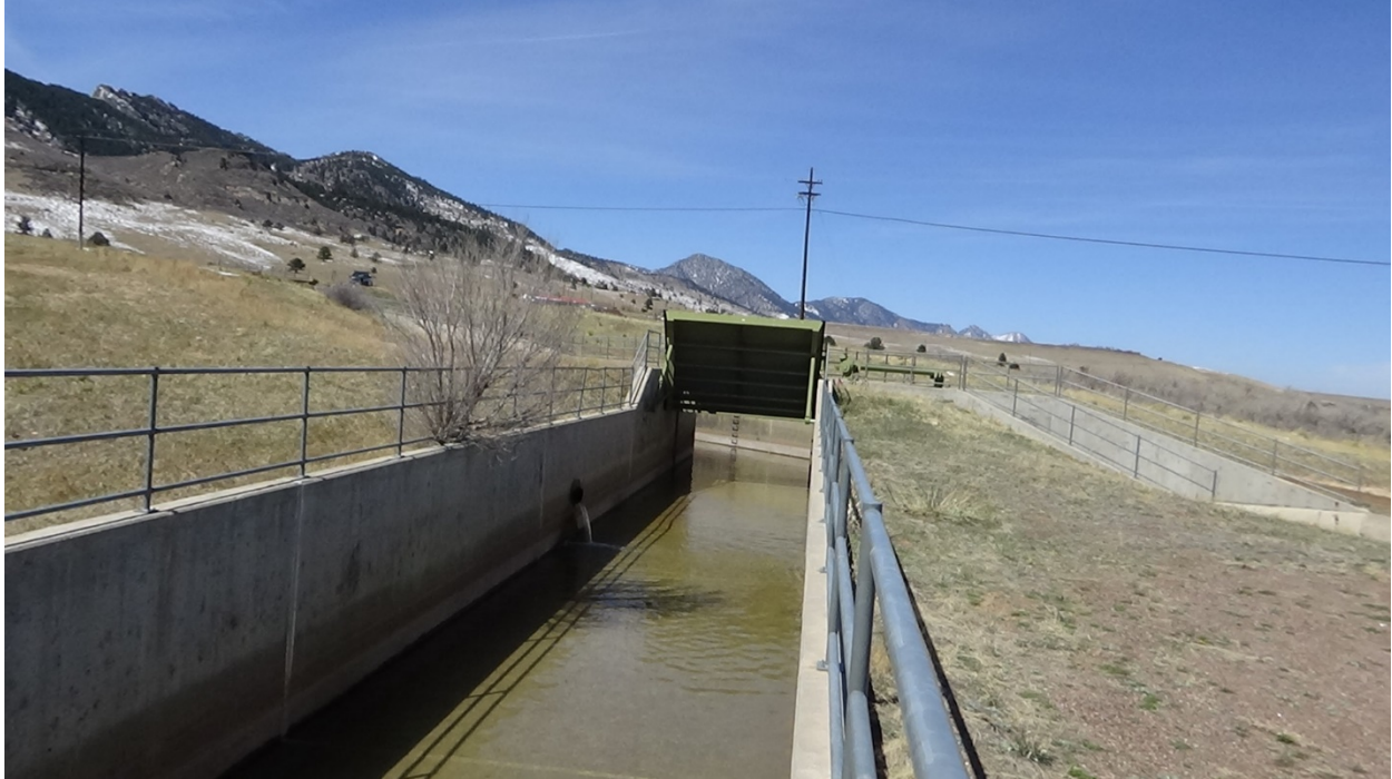
Figure 27 Zone A flume and regulating gate, looking upstream.
