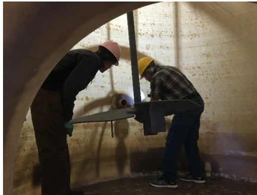
Figure B-2.—Visual inspection of the acid tank interior
