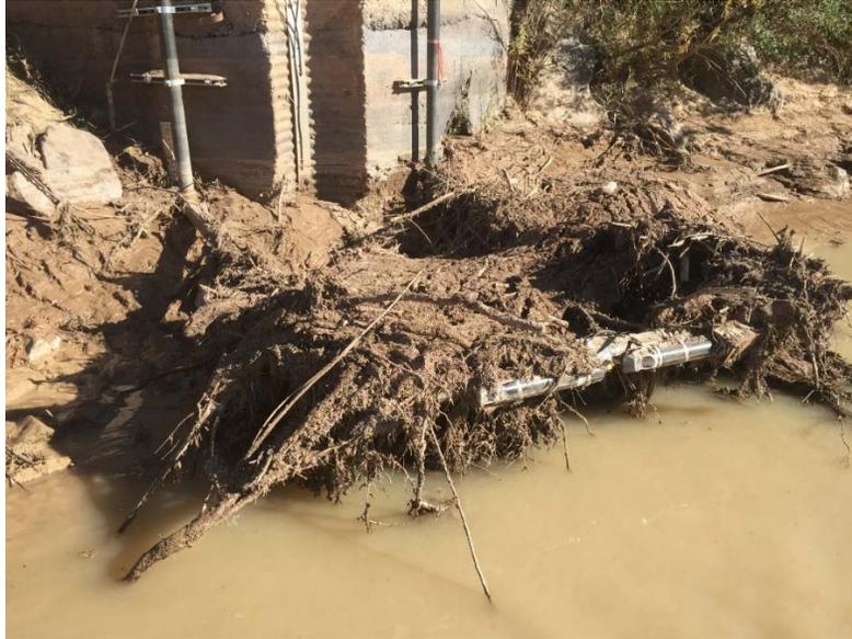
**Figure 17. Debris and sediment left from storm surge on uncontrolled tributaries upstream of the USGS San Acacia gaging station. This material was subsequently cleared away by NMWSC. Photograph taken by T. Austring, NMWSC, on October 13, 2016.**
