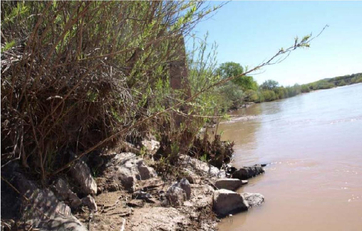
Figure 5. USGS San Acacia gaging site, looking upstream from the old stilling basin structure. Rock used to stabilize bank. Note debris caught in the vegetation above the rock toe. Photograph taken by J. AuBuchon on April 20, 2016.
