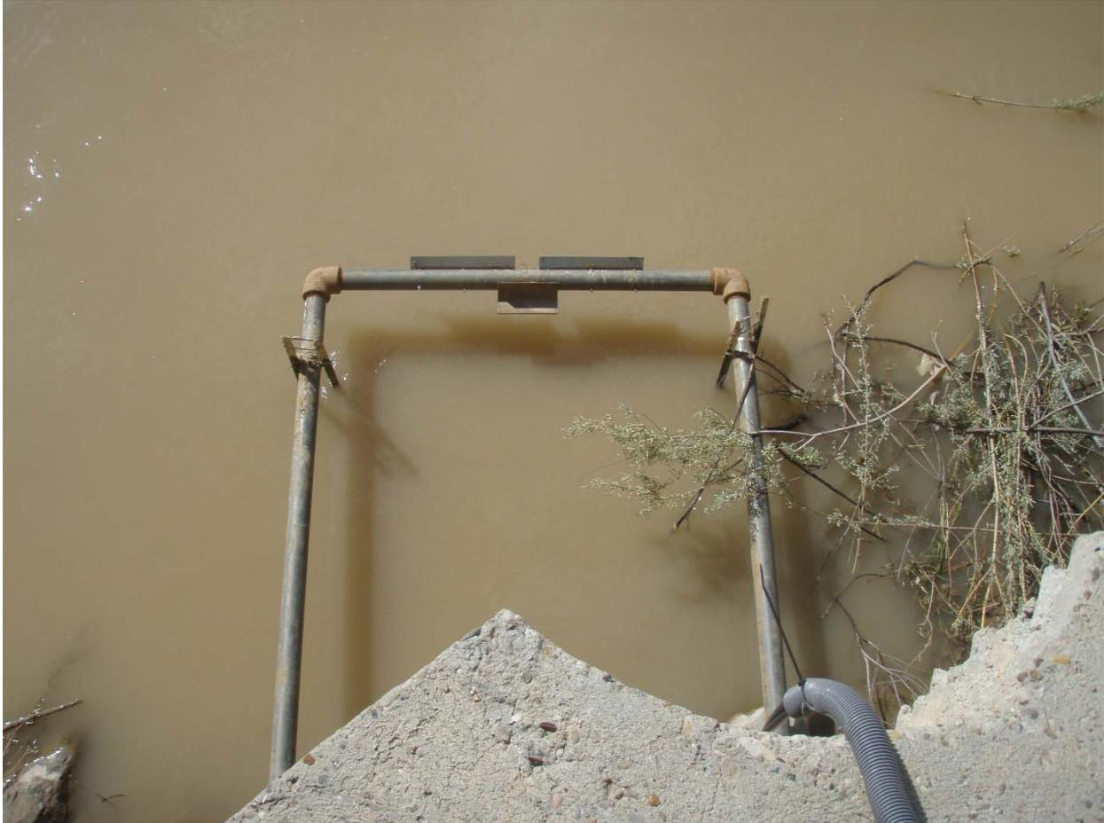
**Figure 10. Installation of acoustic mounting structure at USGS San Acacia gaging station, looking down from top of old stilling basin structure. Photograph taken September 2016 by J. AuBuchon.**
