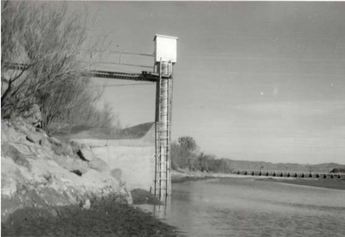
**Figure 3. USGS Gaging Station at San Acacia circa 1953, looking upstream. This site was used as the gaging location from 1953 through 1965, when due to settlement of the abutment the location was discontinued. In 1990 the old well house structure was officially removed, leaving only the abutment (Survey 2012).**
