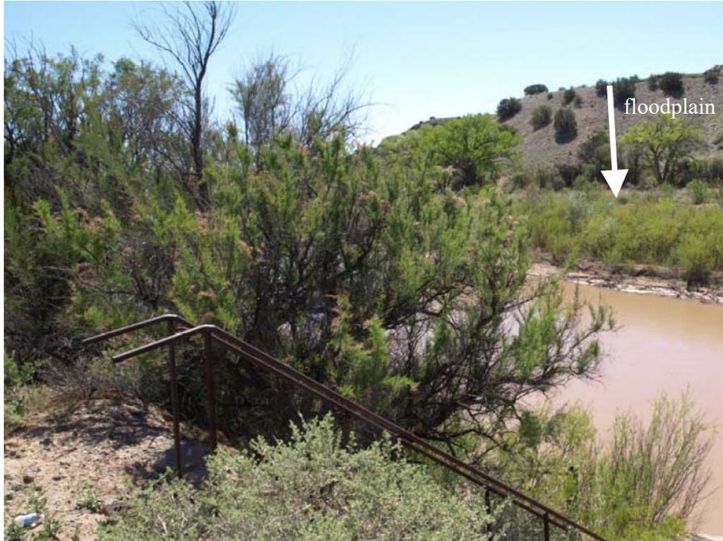
**Figure 7. USGS San Acacia gaging site, looking upstream from the old stilling basin structure from top of right bank. Floodplain on left bank (see arrow) has limited vegetation, indicative of infrequent inundation. Photograph taken by J. AuBuchon on April 20, 2016.**
