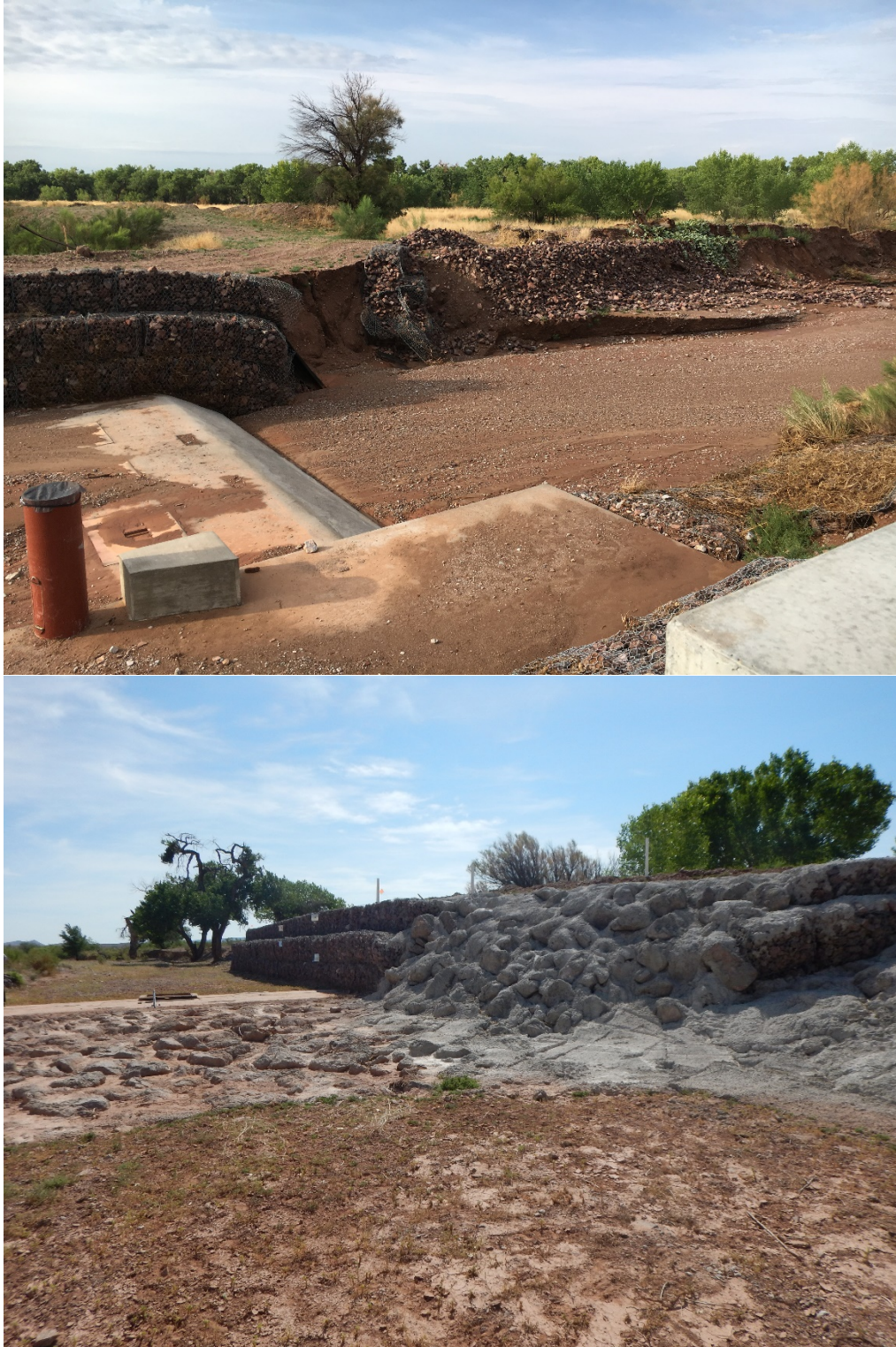
Figure AA- 9 The July 26 th , 2018 was estimated to be a 25-year return interval storm (Lampert and Everetts, 2018). A 'turndown' section of the concrete sill was designed to protect the facility from a headcut propagating from the downstream, which is exactly what happened during this storm (top). The gabion baskets on the left bank were damaged, and the AAO provided a grouted riprap fix (bottom).
