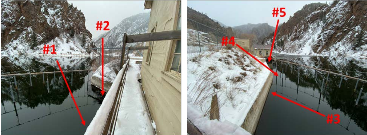
Image 7. The five different locations where structure-to-water potential were measured are shown in the photos.
