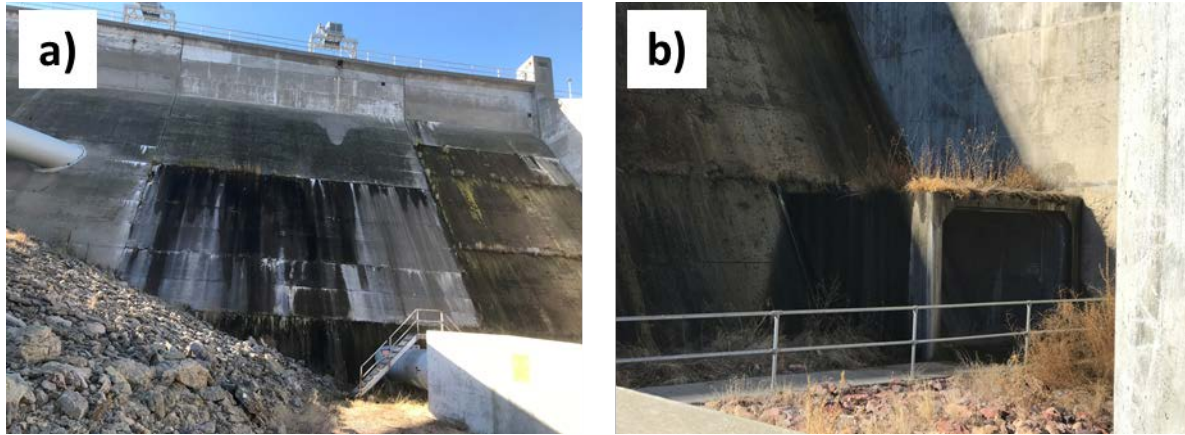
Image 13. Ice formation at Angostura Dam can lead to damage of the discharge pipe shown on the bottom of a) as well as damage to the entrance area shown in b). This also could lead to a risk of injury to dam personnel.
