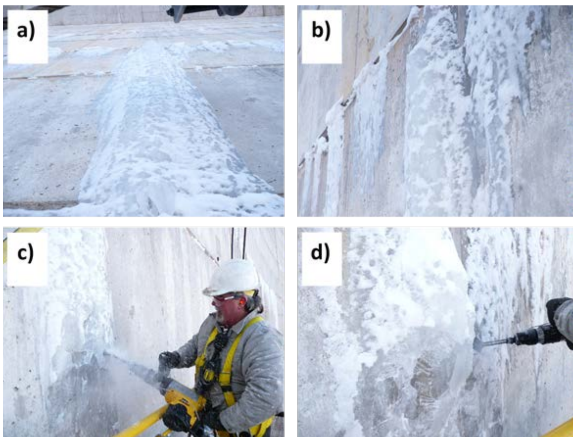
Image 17. Ice formation on the downstream face of the dam caused by water leakage at the lift lines as shown in a) and b). As shown in c) and d) the ice must be manually removed with a chipper.
