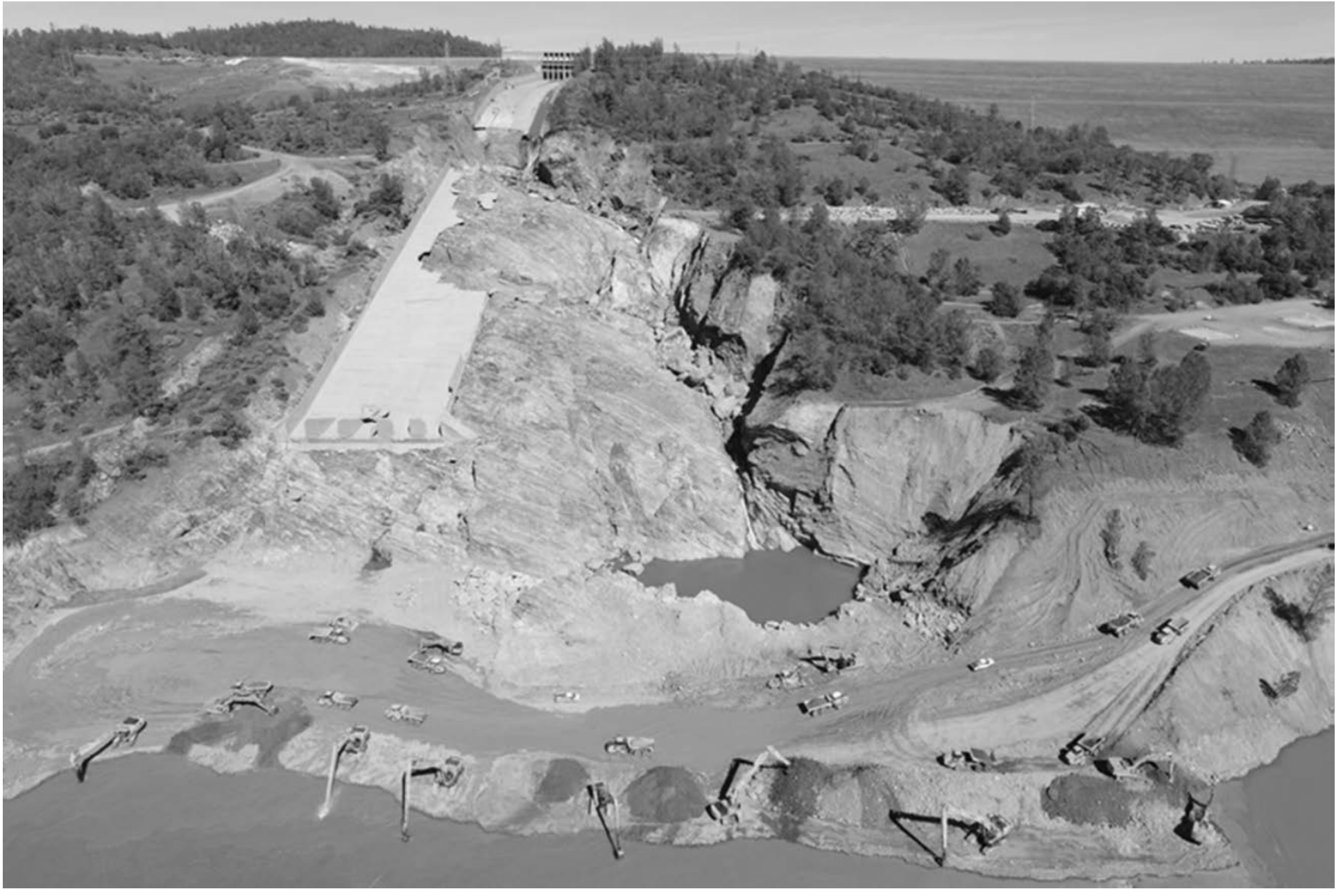
Figure 2. — Ultimate damage at the Oroville Dam service spillway in May 2017 (DWR photo; reprinted from IFT 2018, with permission).
