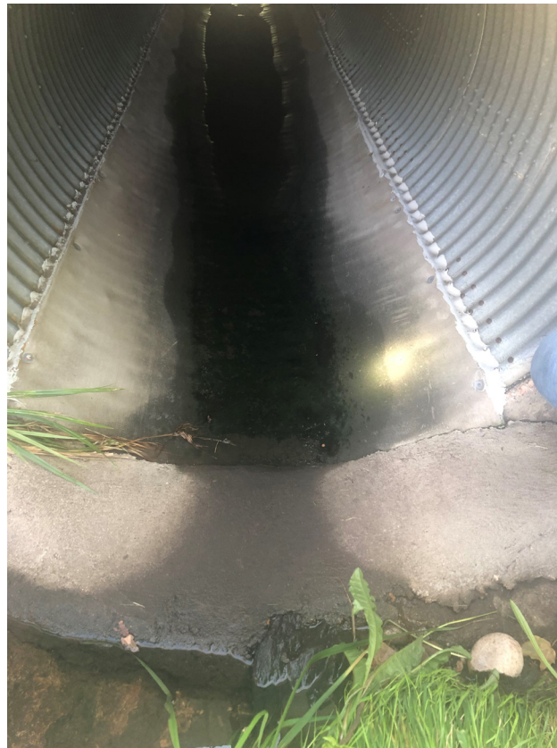
Concrete Cloth™ used to repair corrugated metal pipe.
