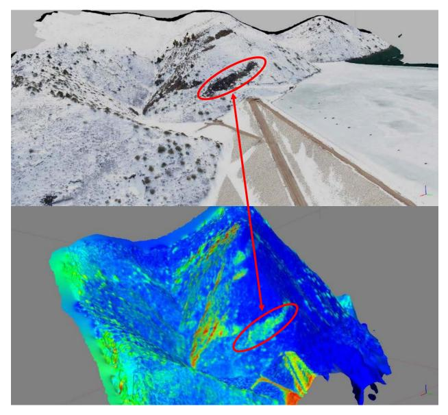
Figure 23.—Comparison of the optical (top) and IR (bottom) 3D models of the north-facing, right abutment at Ridges Basin Dam, Colorado. Note the bare earth and correlating hot spots.
