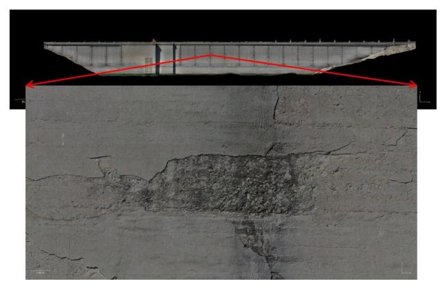
Figure 26.—Elephant Butte Dam, New Mexico, upstream face orthomosaic (above) and example of resolution. Note the aggregate visible in the spall that is approximately 3 feet long (inset).
