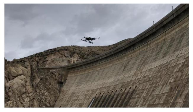
Figure 33.—Intel's Falcon 8+ UAS collecting inspection data at Arrowrock Dam, Idaho.
