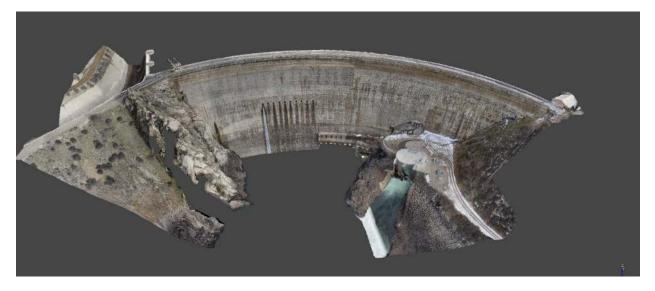
Figure 34.—The meshed model of Arrowrock Dam, Idaho, with a photorealistic texture captured by Intel's Falcon 8+ UAS.
