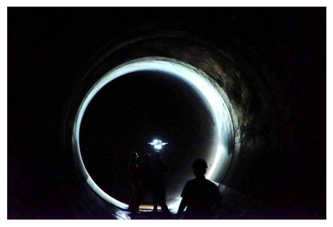
Figure 30.—Testing a tunnel inspection UAS at Glen Canyon Dam, Arizona.
