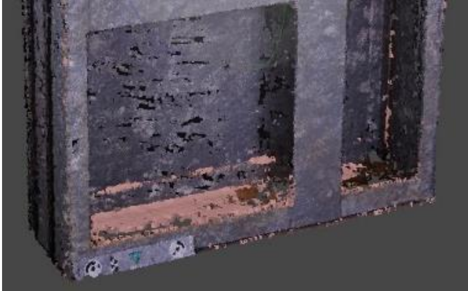
Figure 16: Feature extraction for corrosion in lower compartment of gate with corrosion highlighted as pink; the analysis could not differentiate between rusting staining and fouling.
