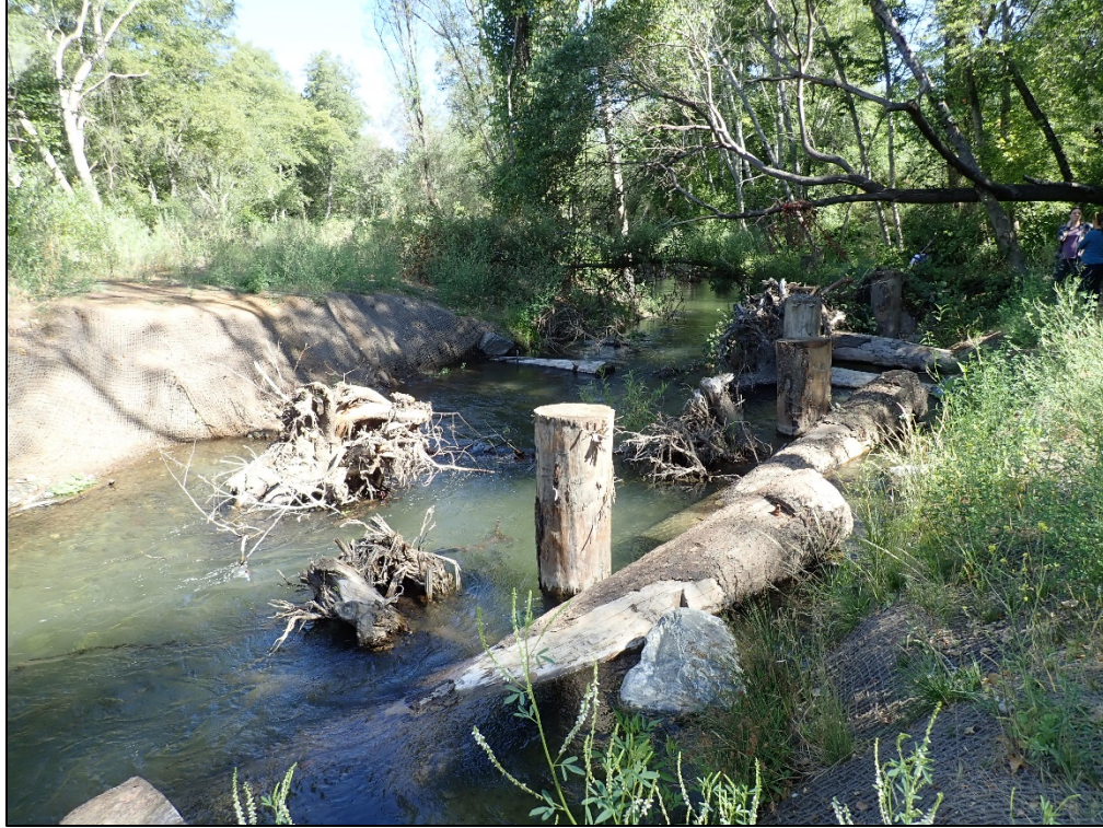
Figure 6. Example large wood structure installations at City of Healdsburg site. Flow at time of site visit was 90 cfs.
