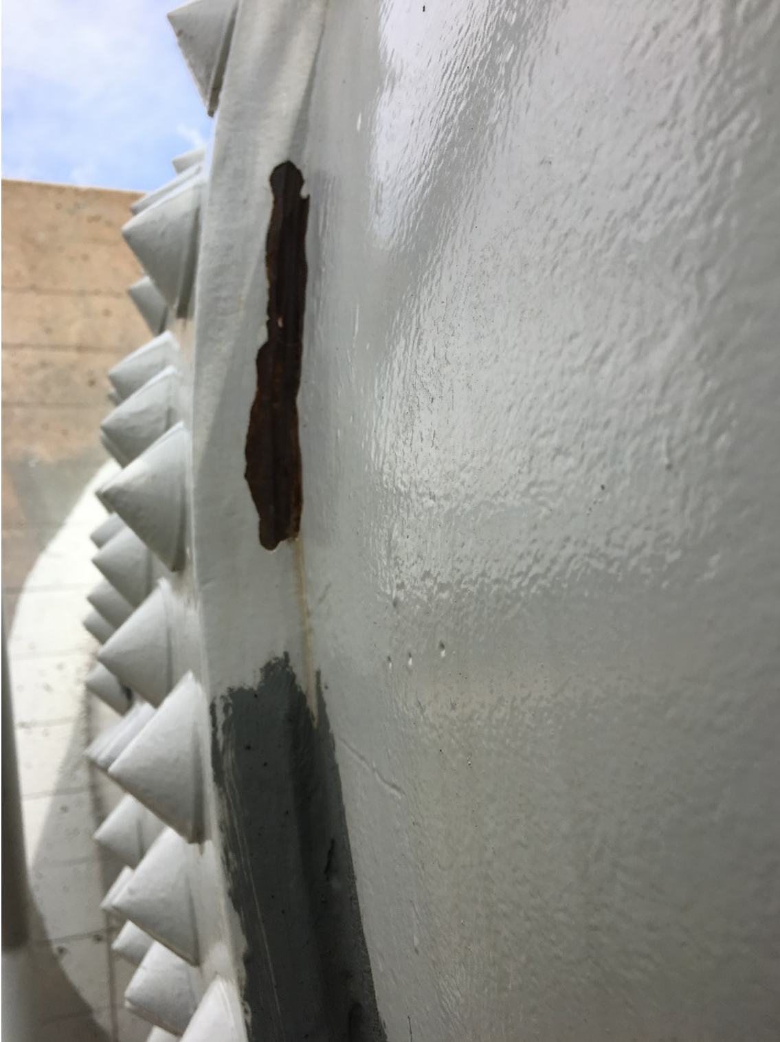
Figure 7. Adjacent to the anodic alkyd spot repair (lower area) another area has cracked and spalled (upper area).
