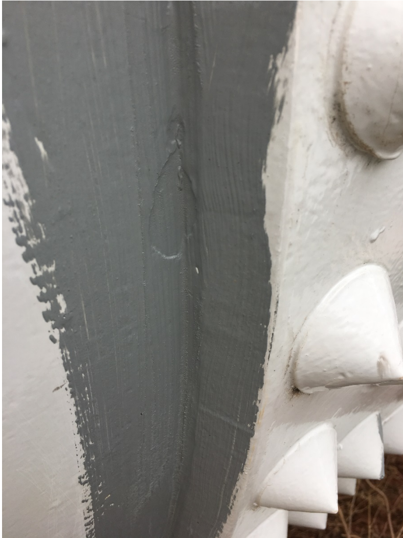
Figure 8. A successful anodic alkyd spot repair after 6 months.
