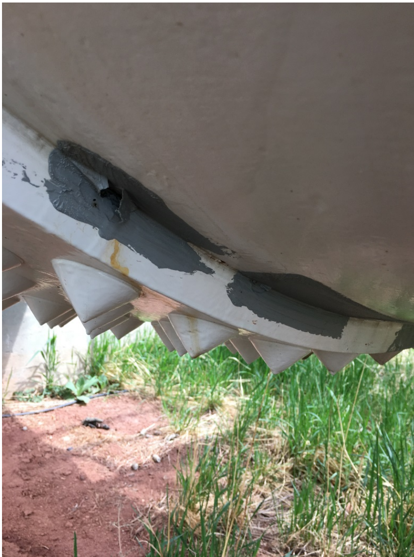
Figure 5. Anodic alkyd spot repairs after 6 months exposure, some areas had cracked coating.
