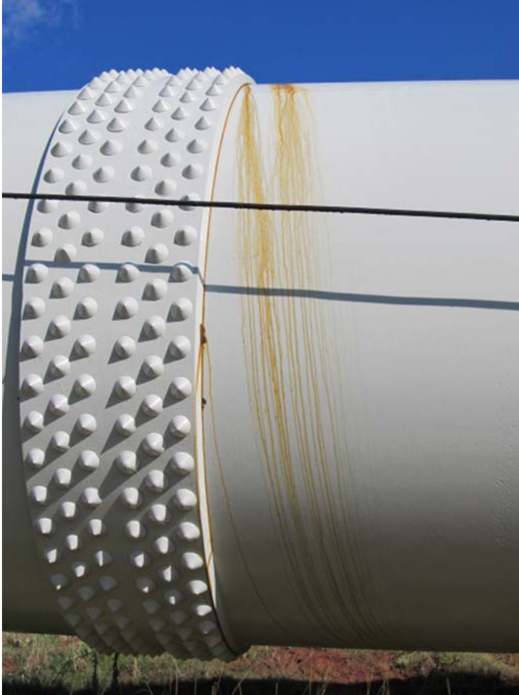
Figure 1. Flatiron penstock riveted connection, coating failure at collar due to vibration
