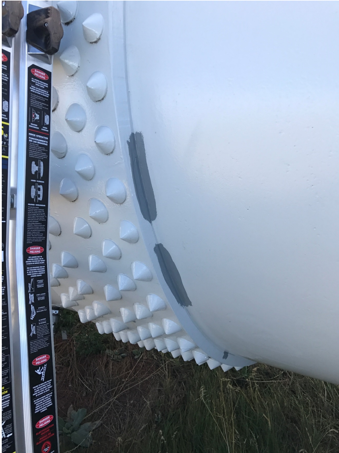
Figure 4. Anodic alkyd spot repairs at the steel collar interface.
