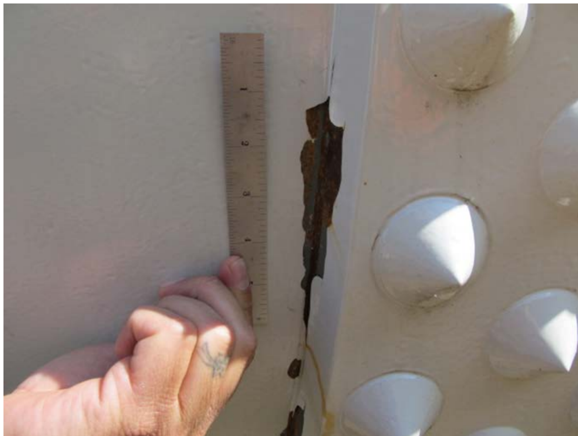
Figure 2. Flatiron penstock riveted connection, closeup of coating failure at collar
