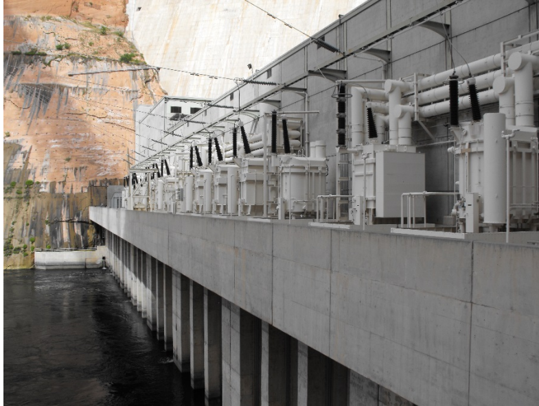
Figure 13 - GSU Power Transformer Deck
