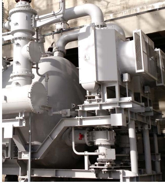
Figure 12 - Gas Blowers on a Gas-insulated Transformer
