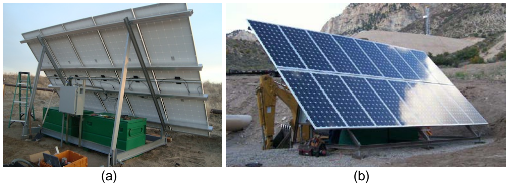
Figure 8.—CP system installed for Chevron Oil with (a) 245 W modules, batteries, and charge controllers in Utah, and (b) 20 A output in Colorado, reproduced from [23]
