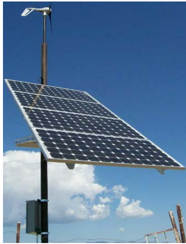
Figure 11.—A CP unit in Wyoming featuring both solar and wind power, reproduced from [23]
