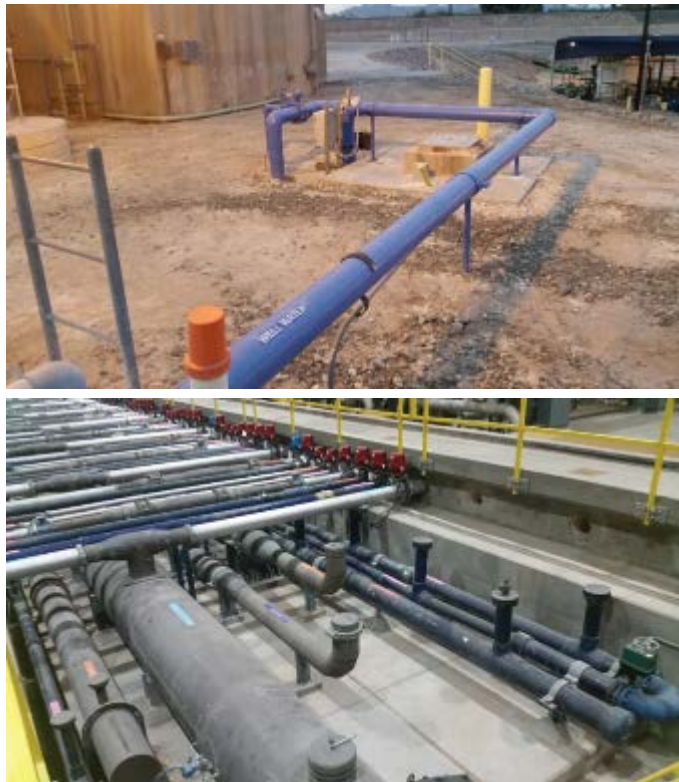
Figure 2. — GRP aboveground pipelines at Yuma Desalting Plant.
