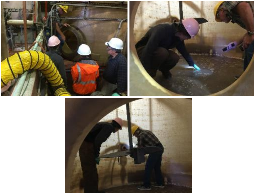
Figure B-2.—Visual inspection of the acid tank interior
