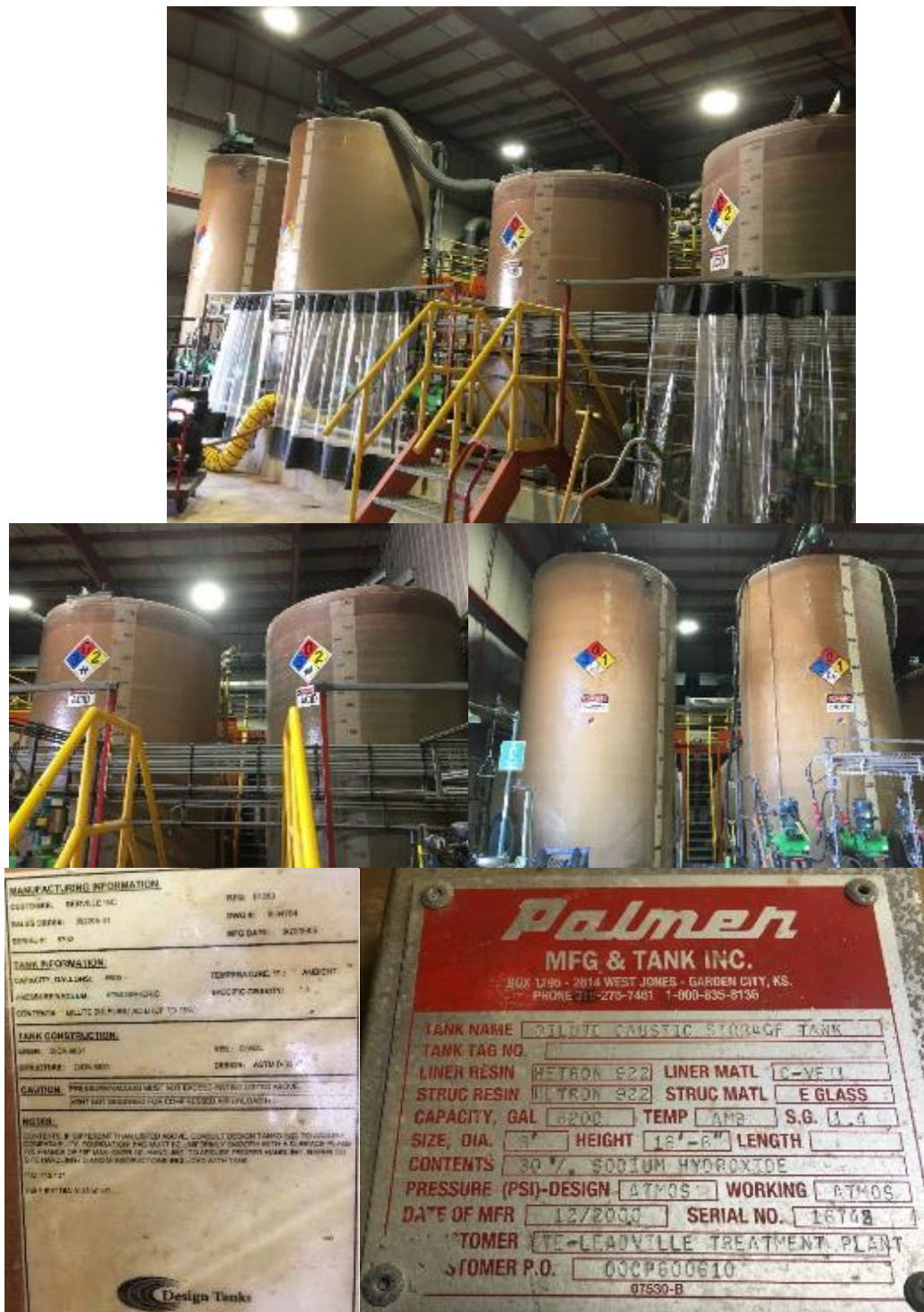
Figure B-1.—Acid and caustic tanks used for water treatment with their manufacturing information
