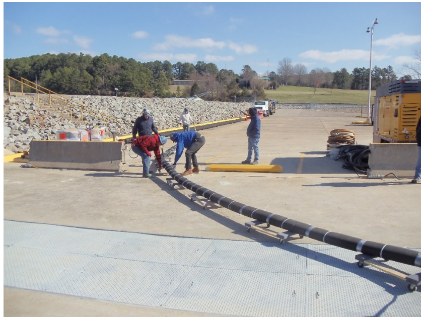
Figure 6 – View showing the waterstop membrane being transported to the core hole via dollies. Note duct tape and zip ties holding the collapsed shape.
