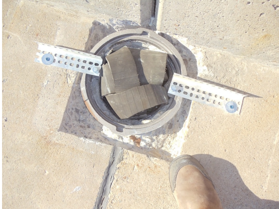
Figure 10 – View showing a previously completed installation. The concrete was cut out to allow installation of the inspection cover (to be filled in with repair mortar at later date). The temporary brackets will be removed after the repair mortar has set.
