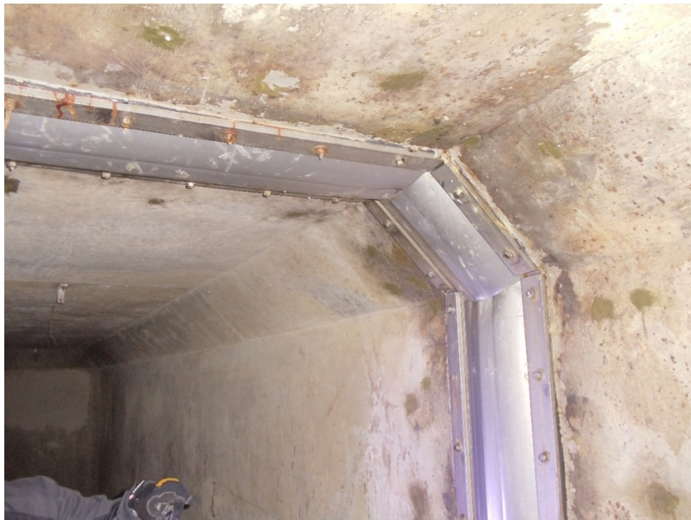
Figure 13 – View showing a waterstop system installed along a contraction joint within the inspection gallery. Note the waterstop is bulged outwards due to the water pressure.
