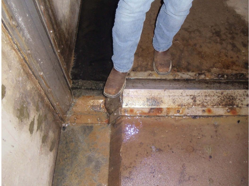
Figure 14 – View showing the bottom portion of waterstop system shown in Figure 11. Note the waterstop is bulged outwards due to the water pressure.
