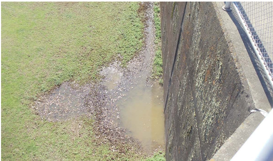
Figure 11 – View showing seepage at the contraction joint prior to insertion of waterstop membrane. Water could be seen exiting face, and percolating upwards from soil.
