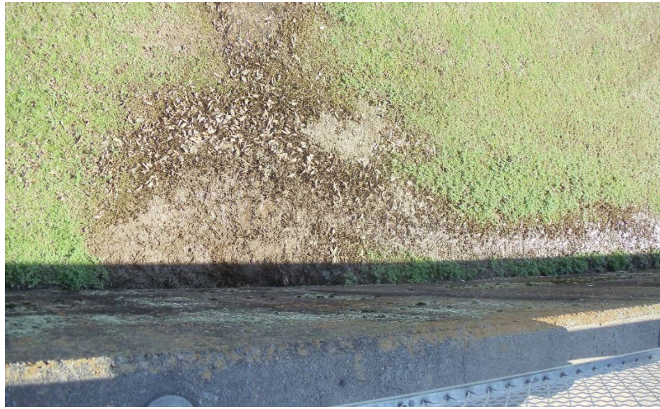
Figure 12 – View showing seepage at the contraction joint after installation and filling of the waterstop membrane.
