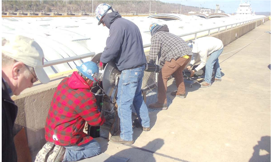
Figure 9 – View of showing the contractor cutting the zip ties as the membrane is inserted. The metal wire is used to cut and remove the duct tape after installation.
