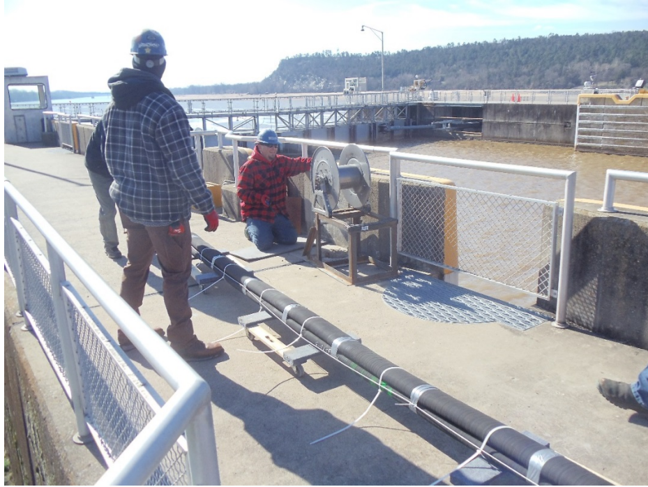
Figure 7 – View showing the waterstop membrane just prior to install into the core hole. Note the spindle used to aid in dropping / guiding the membrane into the core hole.
