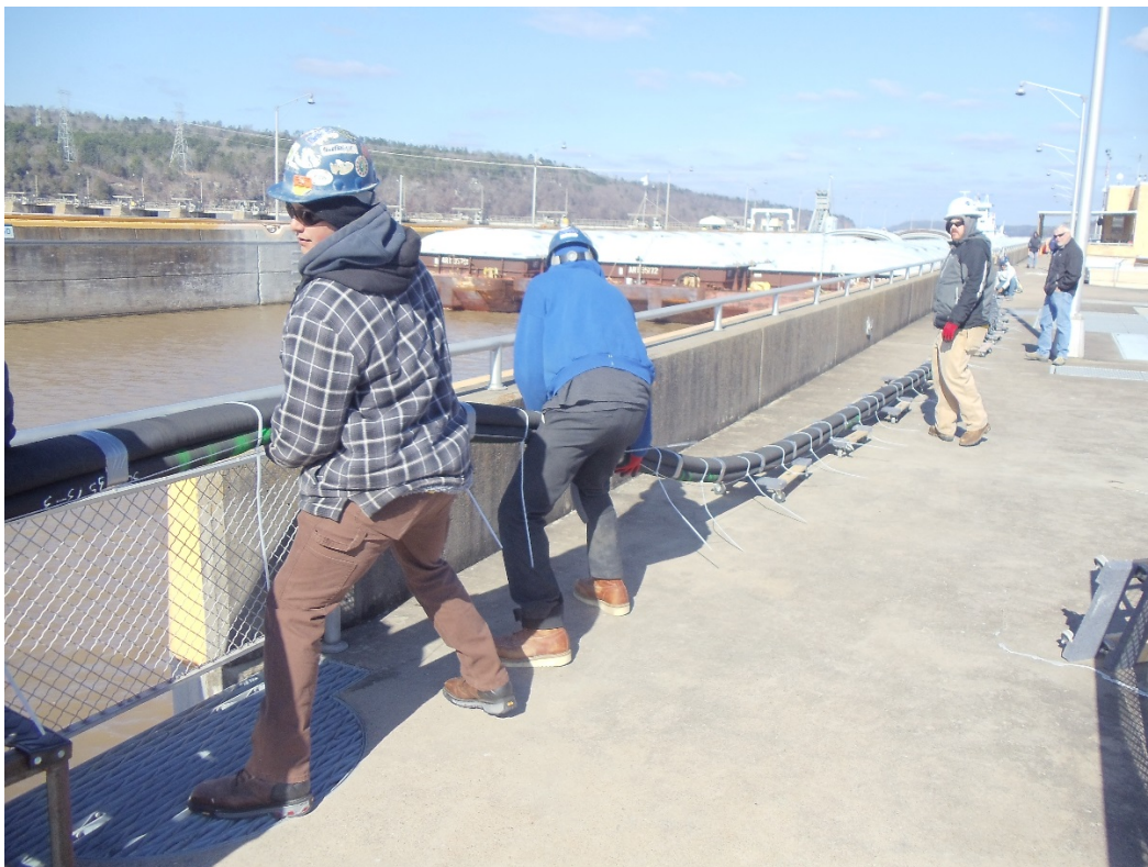
Figure 8 – View showing the manual installation of the membrane into the core hole.
