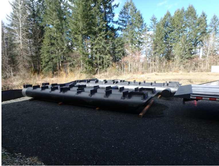
Figure 1. Pontoon barge bases of HDPE 30" diameter pipe prior to assembly and dry fitting.
