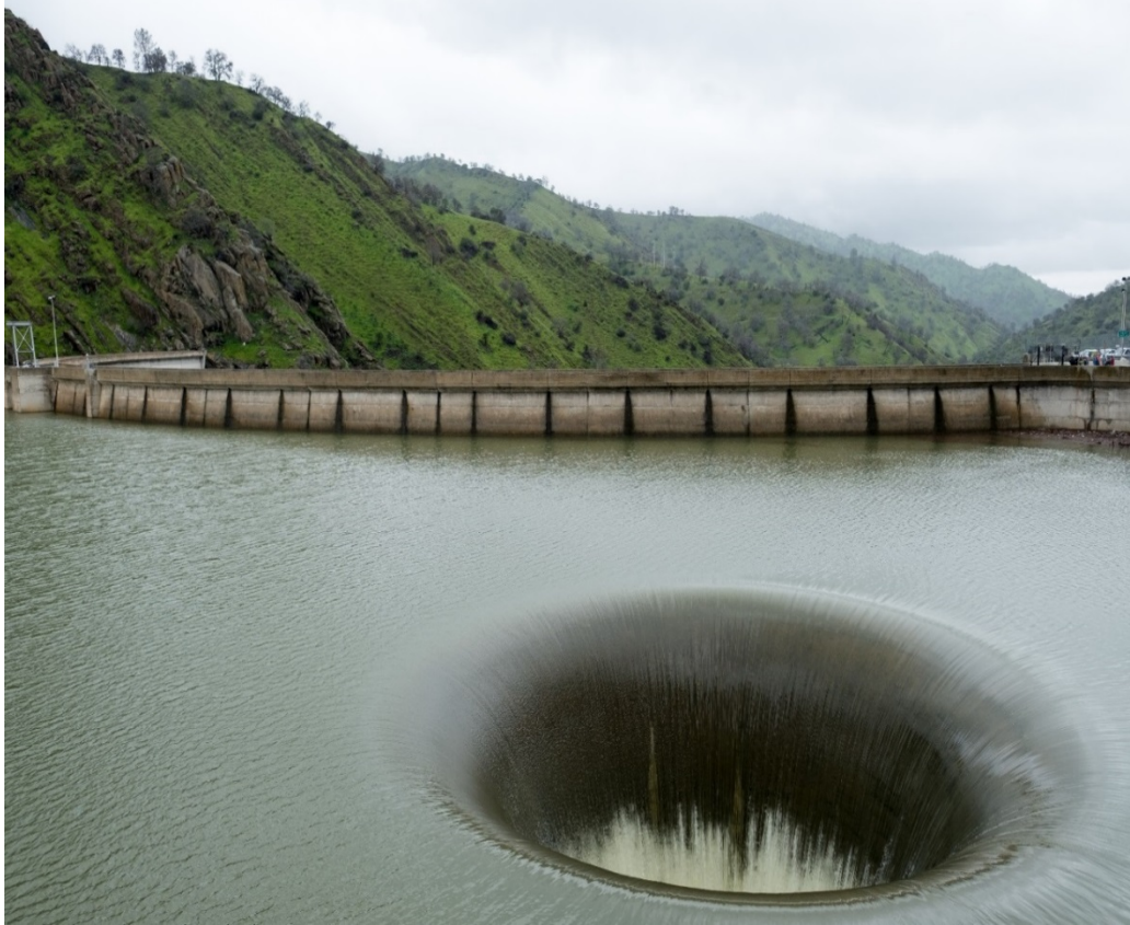
Figure 15. Lake Berryessa and “Glory hole” spillway outlet in Monticello Dam 2
