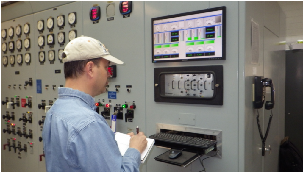
Figure 1. Cavitation display screen from a cavitation monitor at J F Carr powerplant.
