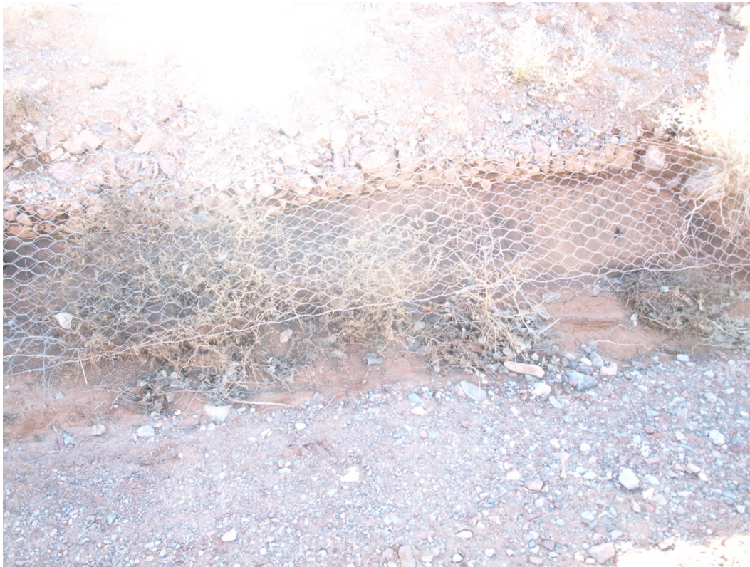
Figure A 1: September 2016 photo of gabionmats eroding at toe on the left bank
