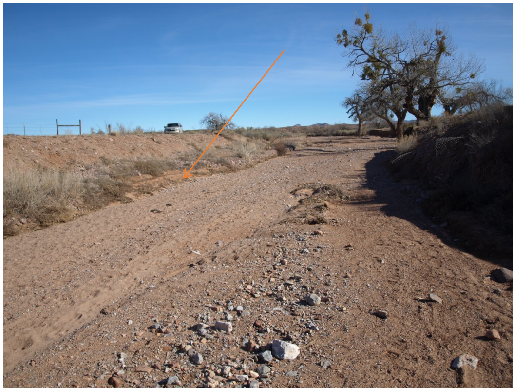
Figure A 2: September 2016 photo of right bank 44' eroded section, looking upstream
