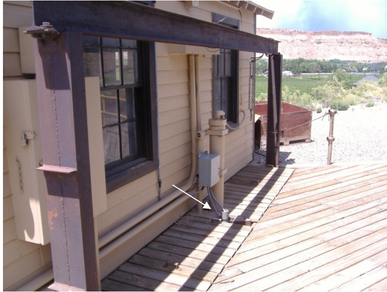
Figure 10. Sensor installation downstream from the OMID hydropower trash rack
