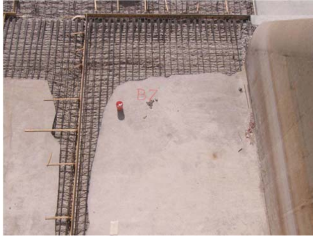
Figure 15. Bay 7 ready for trial concrete placement using concrete containing the Premier Magnesia additive.
