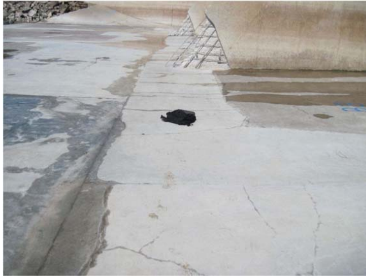
Figure 14. View of shrinkage cracking first observed within one to two weeks of concrete placement.
