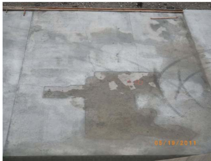
Figure 22. Slab 10 repair made with the trial concrete
