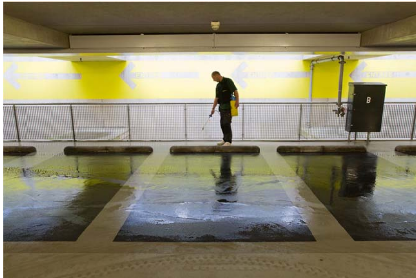
Figure 9. Application of bacterial liquid with hand-carried spraying device
