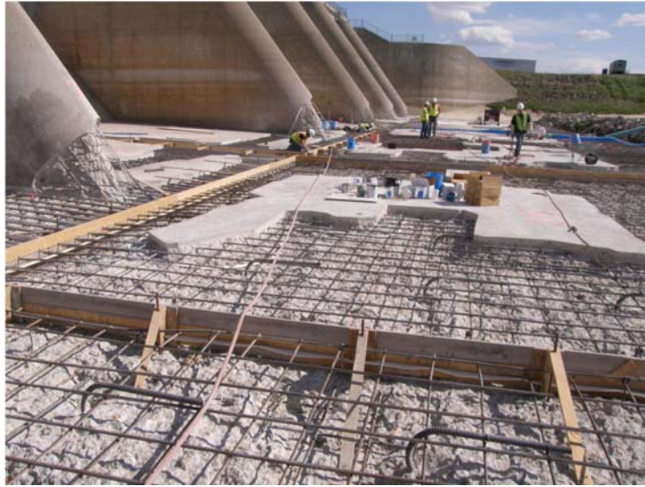
Figure 13. Example of concrete removal with some original concrete remaining
