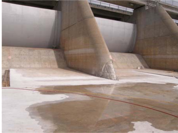
Figure 19. Placement B8/9 made with concrete containing the Premier Magnesia additive.
