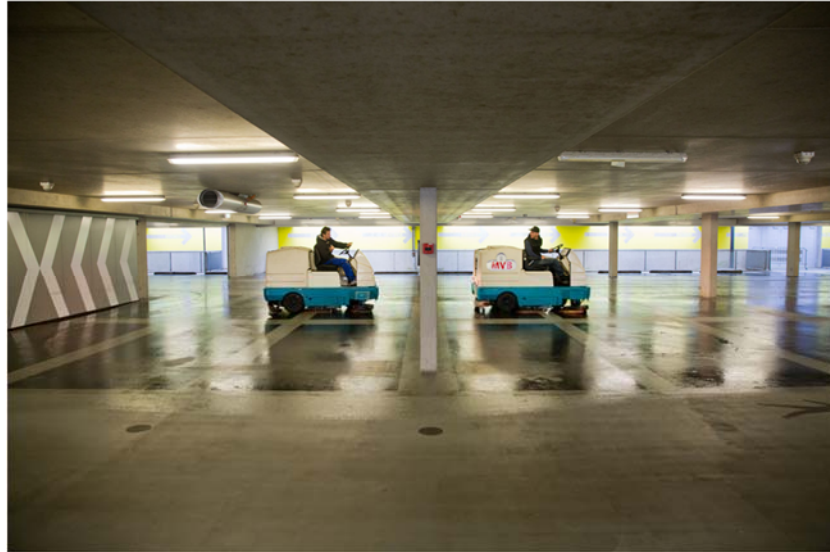
Figure 8. Application of bacterial liquid with scrubbing machines
