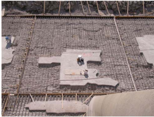
Figure 16. Slab 10 ready for trial concrete placement using concrete containing the Premier Magnesia additive.
