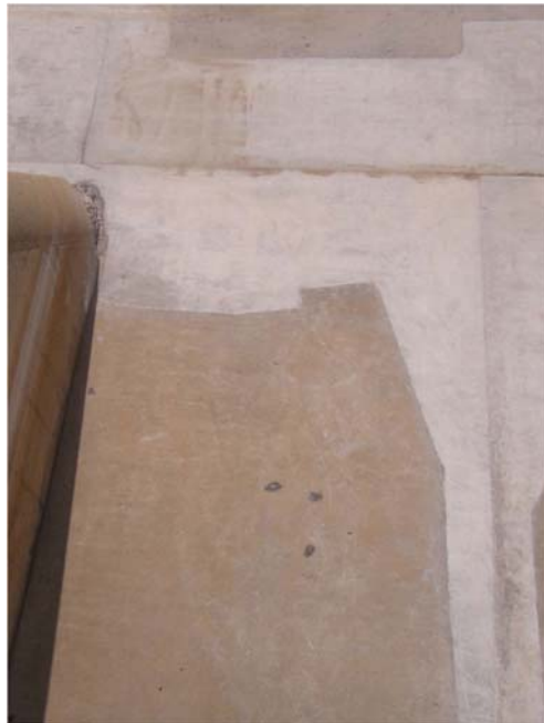
Figure 18. Bay 7 placement made with concrete without Premier Magnesia additive.
