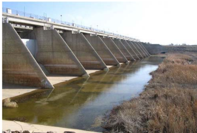
Figure 10. View of approach area of spillway. The soil berm trapped water on the apron, leading to deterioration of the concrete.
