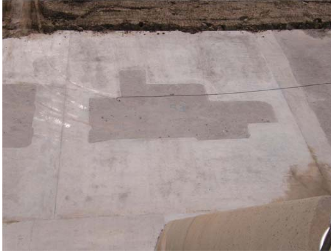
Figure 17. Slab 3 placement made with concrete without the Premier Magnesia additive.
