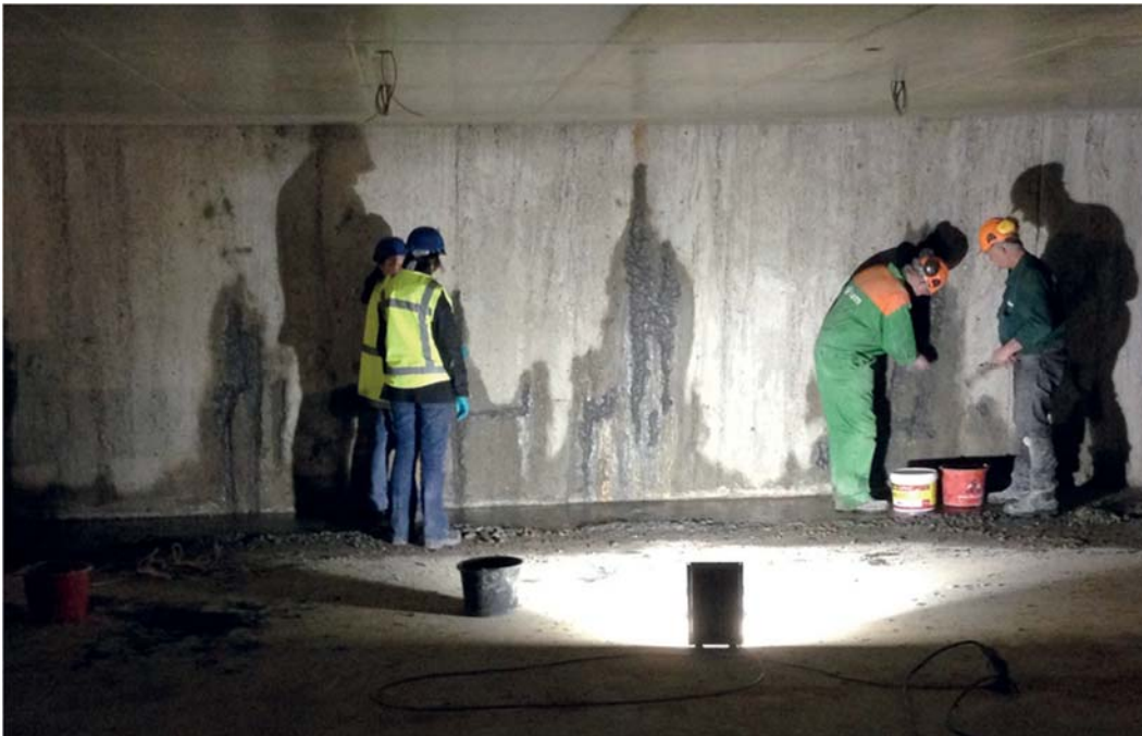
Figure 7. Groninger Forum Diaphragm wall repair with bacterial mortar
