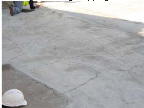
Figure 20. Typical shrinkage cracking mapping and measurement.
