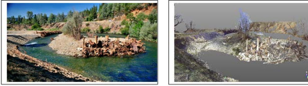
Figure 8. Constructed wood jam on the Trinity River, California – ground photo (left) compared to LiDAR scan point cloud (right)
