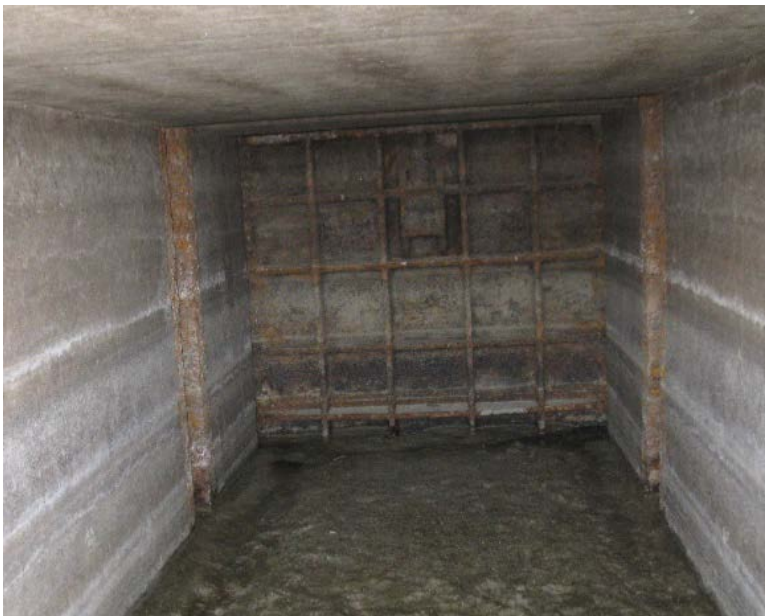
Figure 12. Cast iron slide gate at Kirwin Dam exhibiting significant corrosion along with the stoplog guides.
