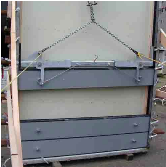
Figure 18. Fiberglass stoplogs used successfully over the past 18 years in numerous applications. [Error! Bookmark not defined.]
