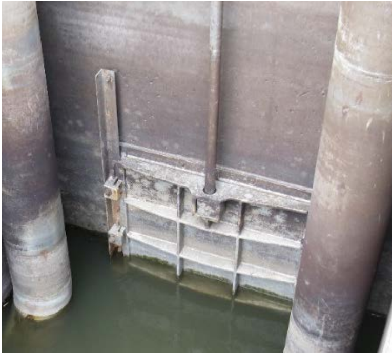
Figure 11. Cast iron slide gate at Enders Dam exhibiting corrosion along the edges of the gate and the stem.
