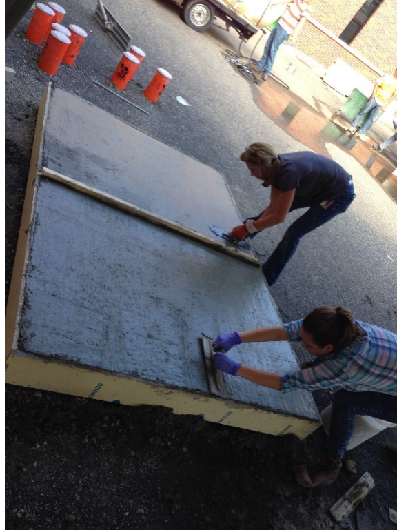
Figure 10. – Surface finishing operation.
