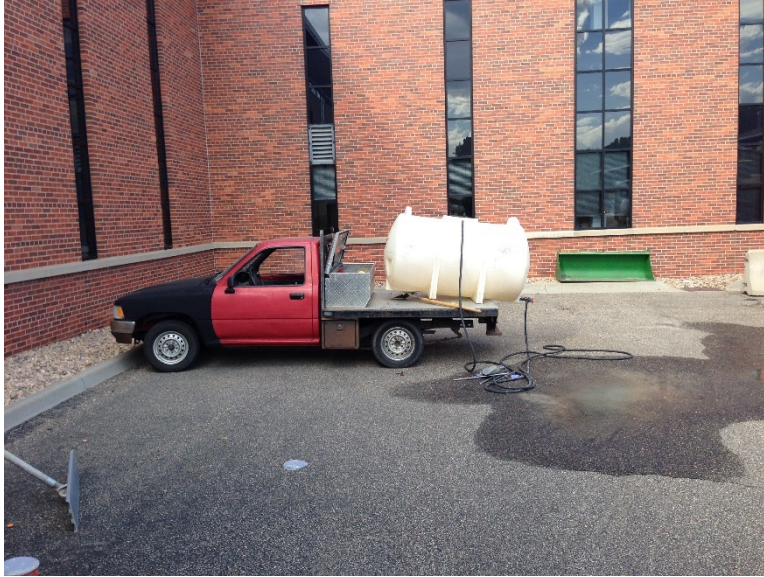
Figure 4. – Mobile water tank used for slab ponding operation.
