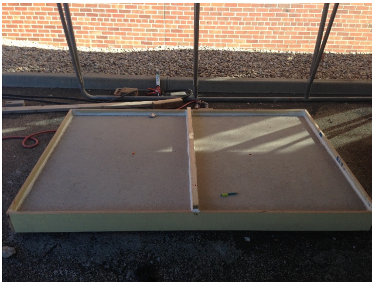
Figure 3. – Formwork installed on one of the cast-in-place 5 by 8 ft test slab prior to overlay placement.
