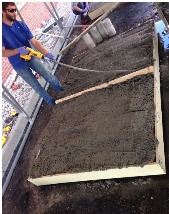
Figure 9. – Vibration of repair/overlay concrete.
