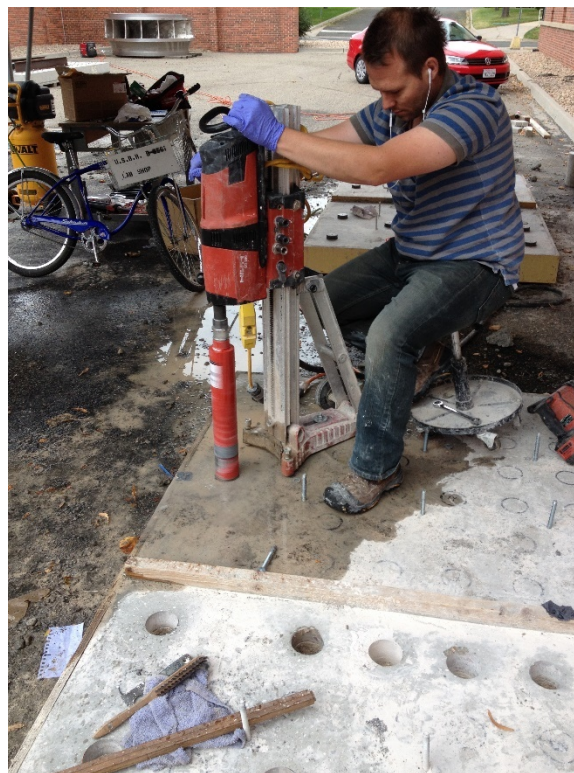
Figure 13. – Core drilling operation.
