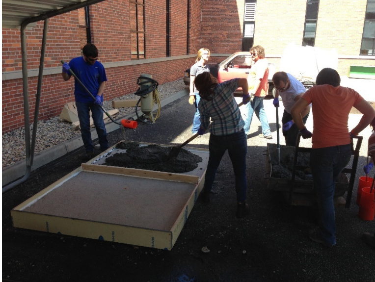
Figure 8. – Placement of repair/overlay concrete.
