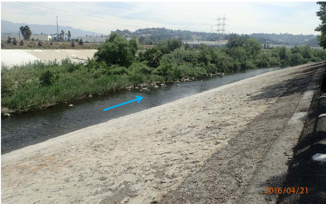
Figure 8. Site 3 looking downstream from the right bank. Note the vegetation growth along the left bank and grouted riprap along the right bank. Photograph taken by Jennifer Bountry (April 21, 2016).
