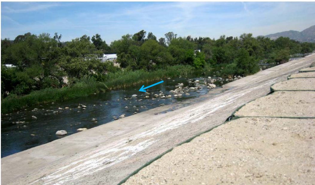
Figure 6. Site 2 looking upstream from the left bank. Note the large cobble sized bed material and vegetation growth near the channel. Sand filled barriers have been temporarily installed along the left bank to raise the bank height due to flooding concerns prior to the El Niño season. Photograph taken by Nathan Holste (April 21, 2016).
