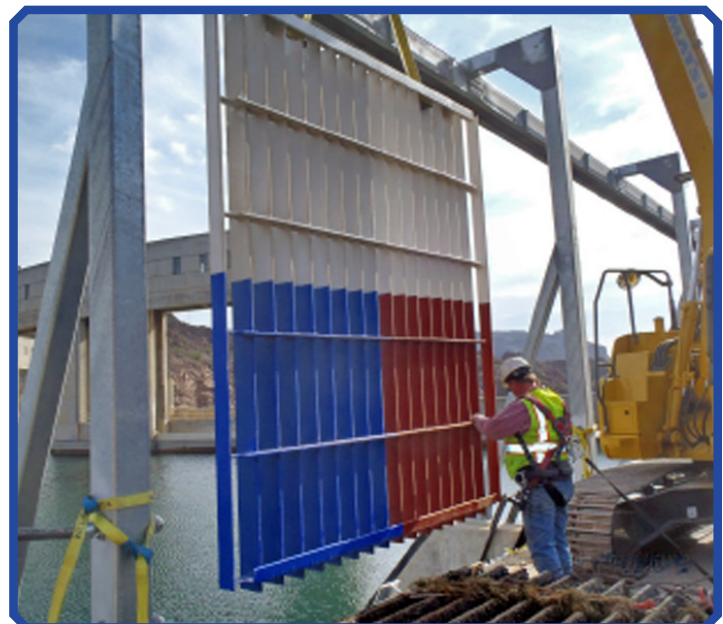
Installing the trash rack panel with four test coatings.
