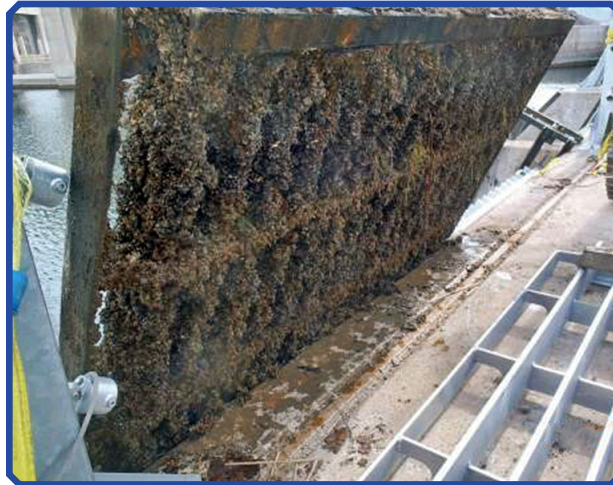
Existing trashrack heavily fouled with zebra and quagga mussels.
