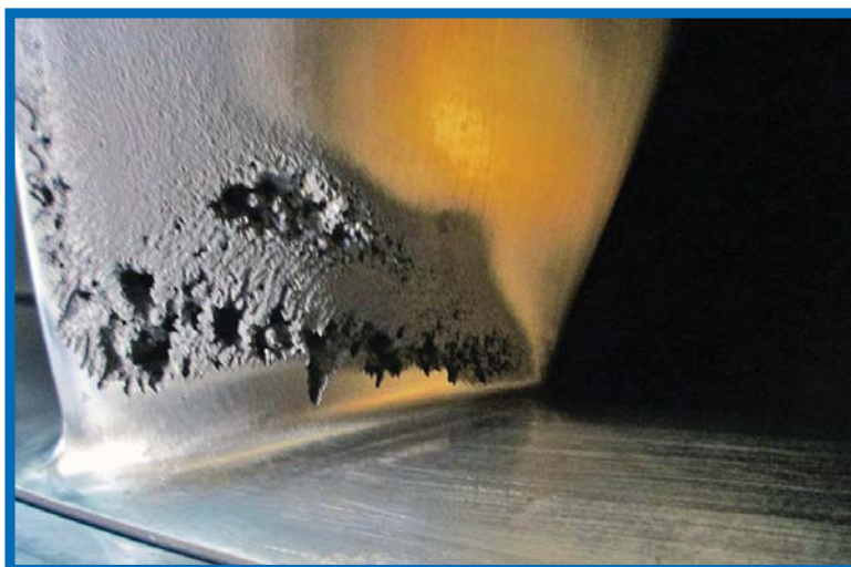
Cavitation damage to a turbine runner blade of J.F. Carr Unit 2 in February 2013. Photograph courtesy of John Germann.
