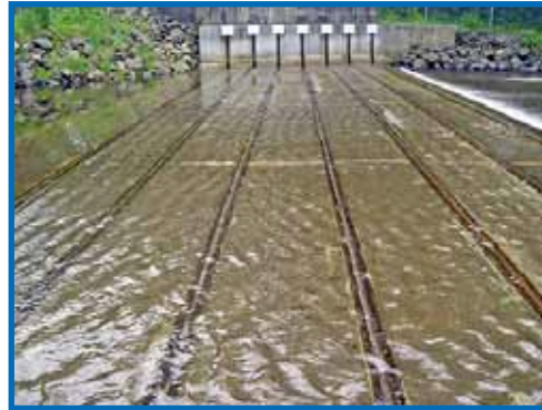
Electric barrier with bottom flush-mounted electrodes at Quinault National Fish Hatchery, Washington.
