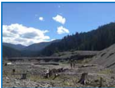
Looking upstream at sediment terraces left behind from dam removal notching and tree stumps where the river has cut tens of feet down through sediment deposits into the pre-dam floodplain.
