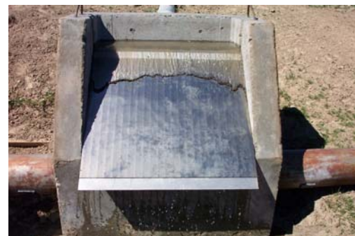
Coanda-effect screen removing fine debris from a piped irrigation delivery
