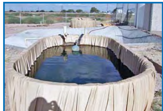
Slowsand filter after being filled up.
