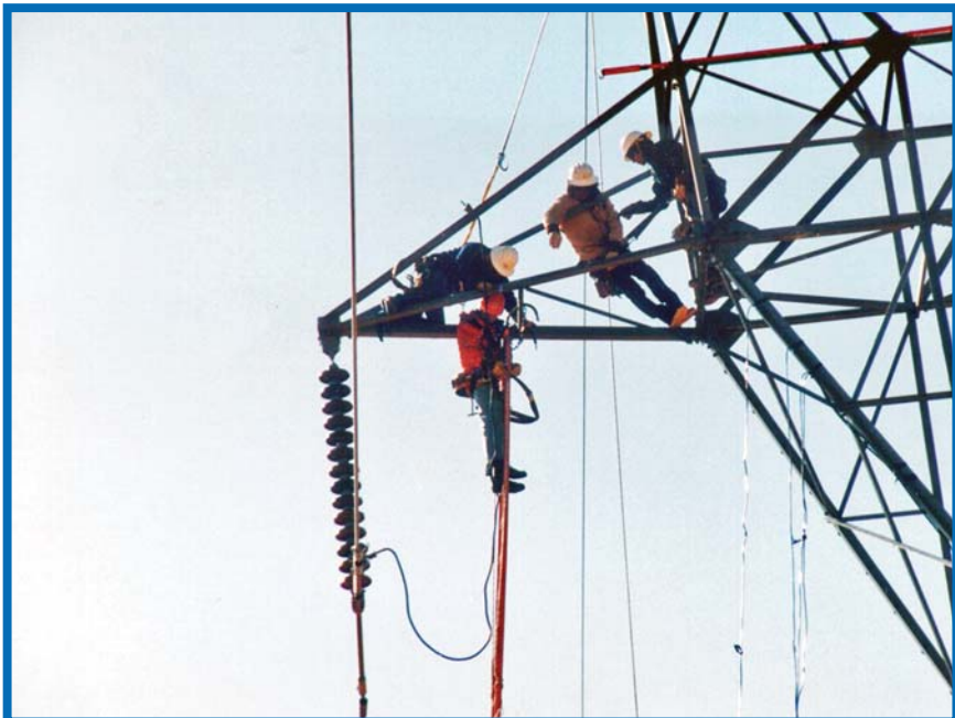
Workers working on high power transformer lines.
