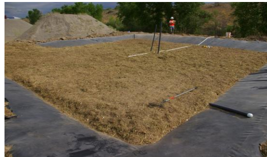
Pilot-scale selenium passive bioreactor cell.
