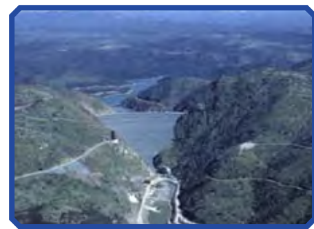
New Melones Dam and Reservoir, California
