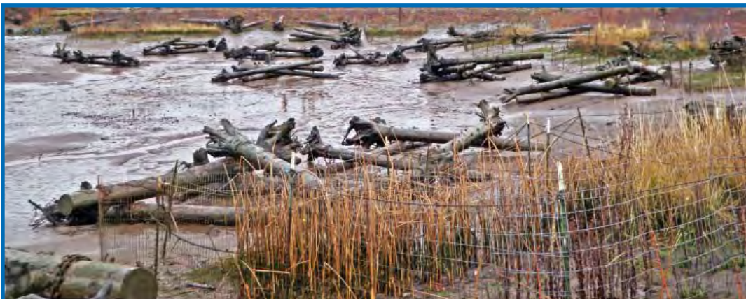
North Wind’s Weir site where King County, Washington, and U.S. Army Corps of Engineers have been placing earth-anchored log clusters in fine-grained soil to improve tidal backwater conditions at an urban site near Seattle that has local cultural significance. Photograph by Connie Svoboda, Reclamation’s Technical Service Center, February 2012.
