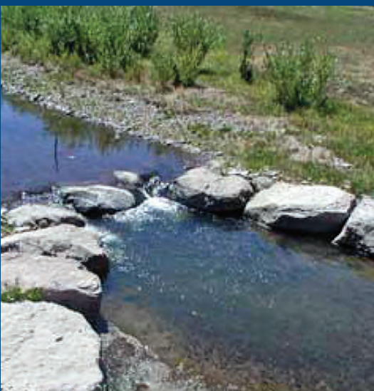
Rock weir structure.
