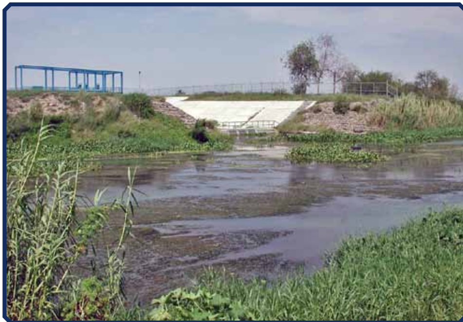
Intake structure blocked by Hydrilla and water hyacinth.
