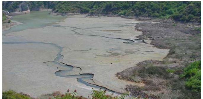
Matilija Dam and Reservoir with extensive sediment deposition in the foreground and the dam in the far upper left corner
