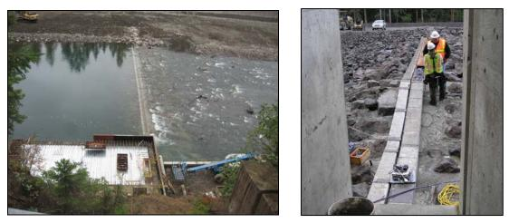
Figure 3. New diversion weir (river km 5.6) constructed across the Elwha River in October 2008. The picture on the right shows the low flow notch during construction. Flow direction in both figures is from left to right.
