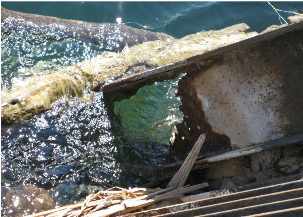
Figure 17.—Parker Dam Trashrack fluctuating water zone, prior to replacement.
