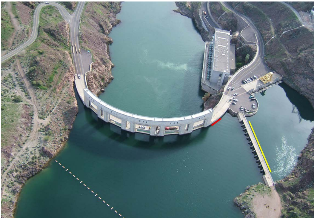
Figure 1.—Aerial photo of Parker Dam, CA. The red line indicates the location where the plates were placed, and the yellow line indicates where the grates were placed.
