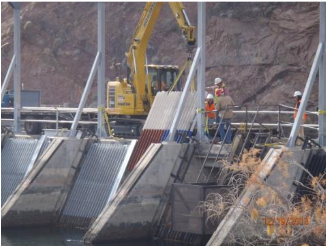
Figure 5.—Installation of the new foul-release coated panel.
