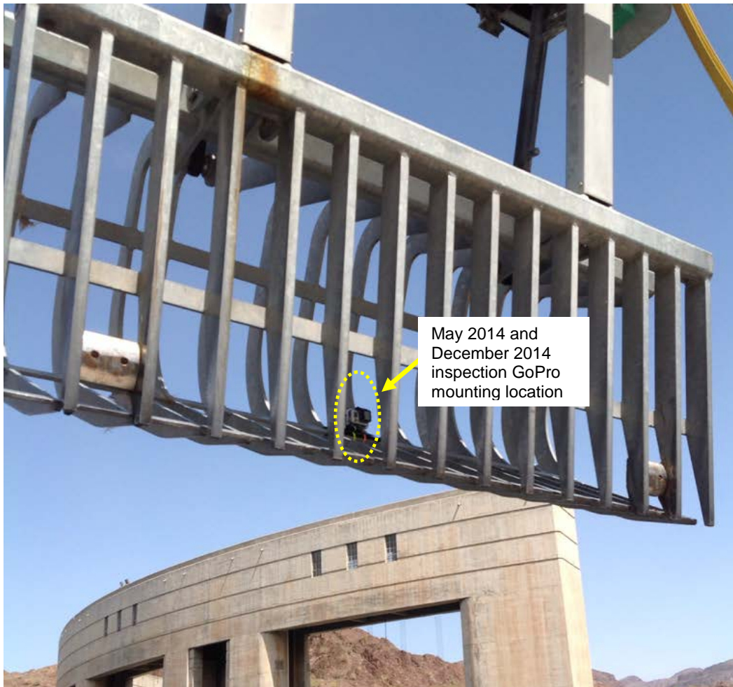
Figure 11.—Trashrack cleaner with GoPro camera mounted.
