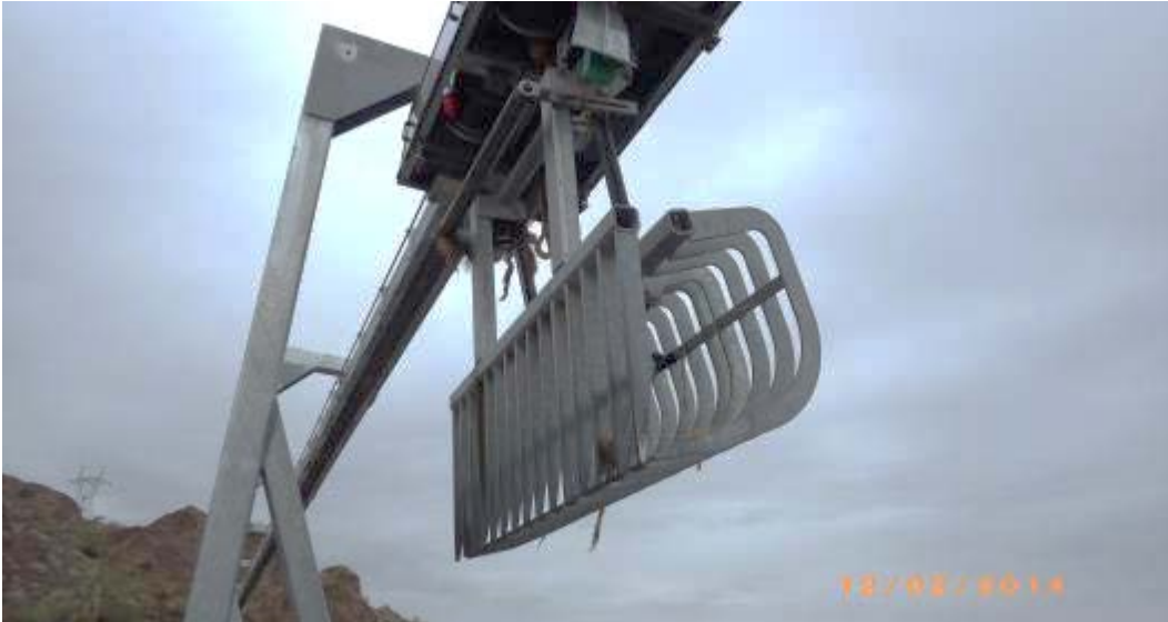
Figure 12.—Trash rake has a roller in the back and two guides on the bottom of the rake.
