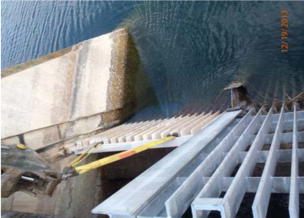
Figure 6.—Installation of the new trashrack panel.
