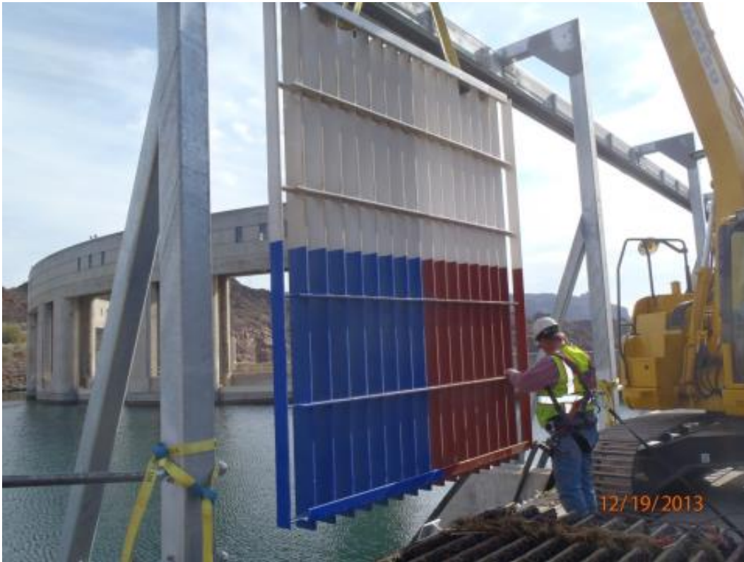
Figure 4.—Installation of the new trashrack panel.
