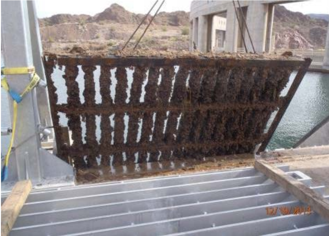
Figure 2.—Existing trashrack, view looking east.
