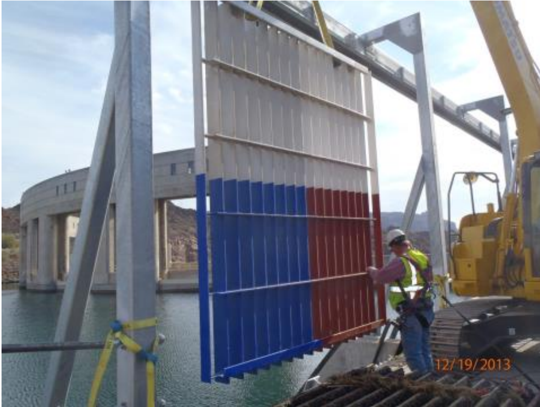
Figure 4.—Installation of the new trashrack panel.
