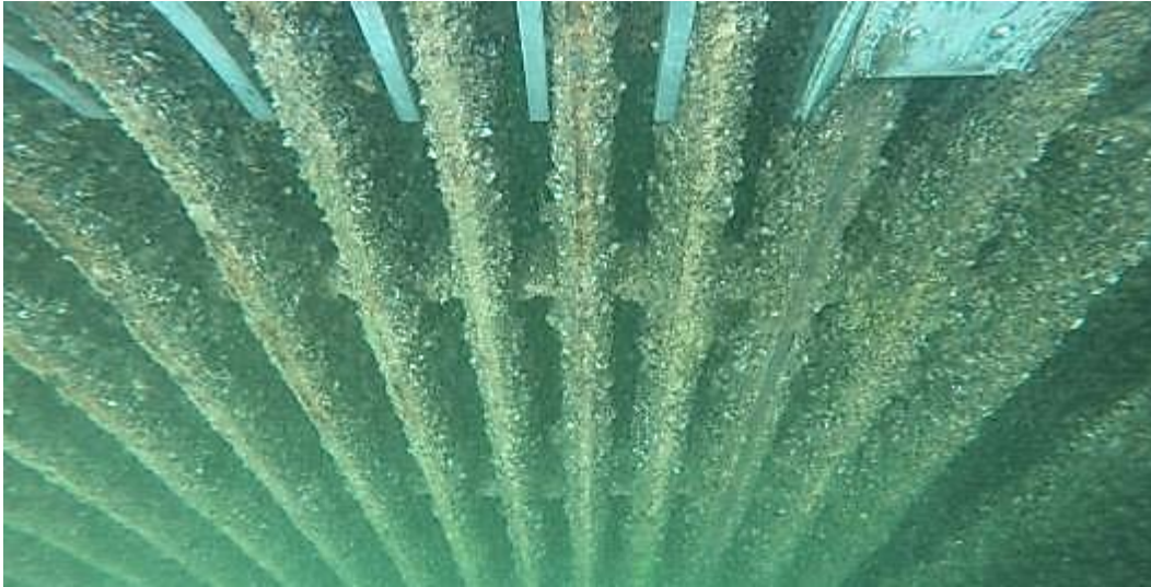
Figure 14.—Existing coal tar enamel coated trashrack.
