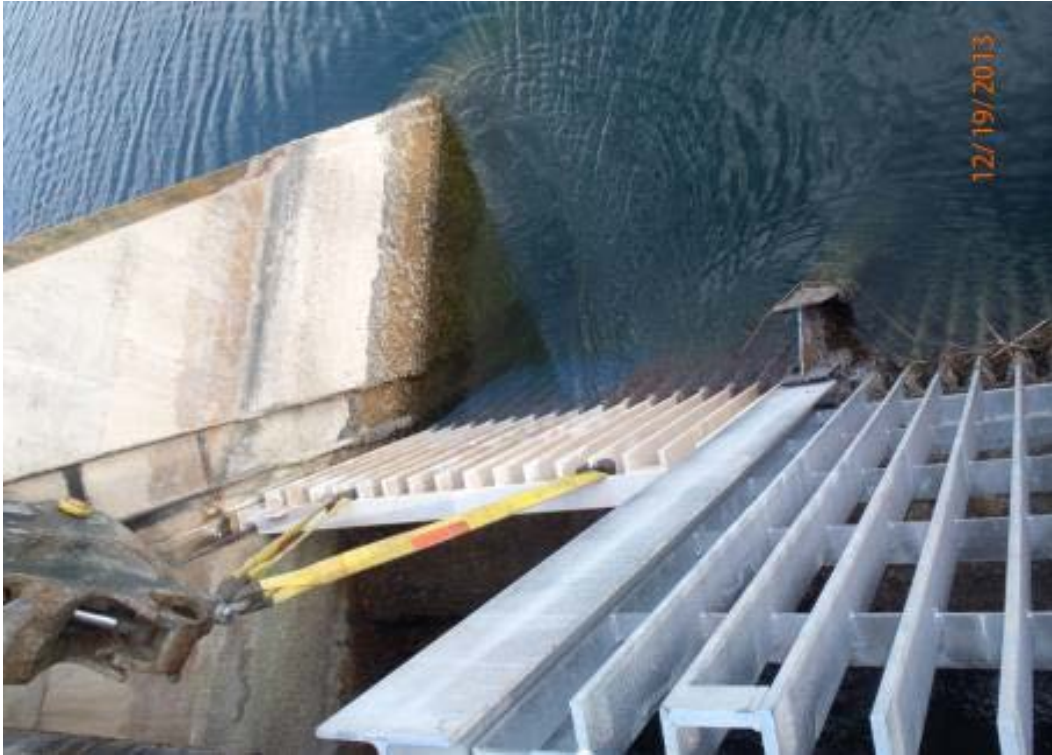
Figure 6.—Installation of the new trashrack panel.
