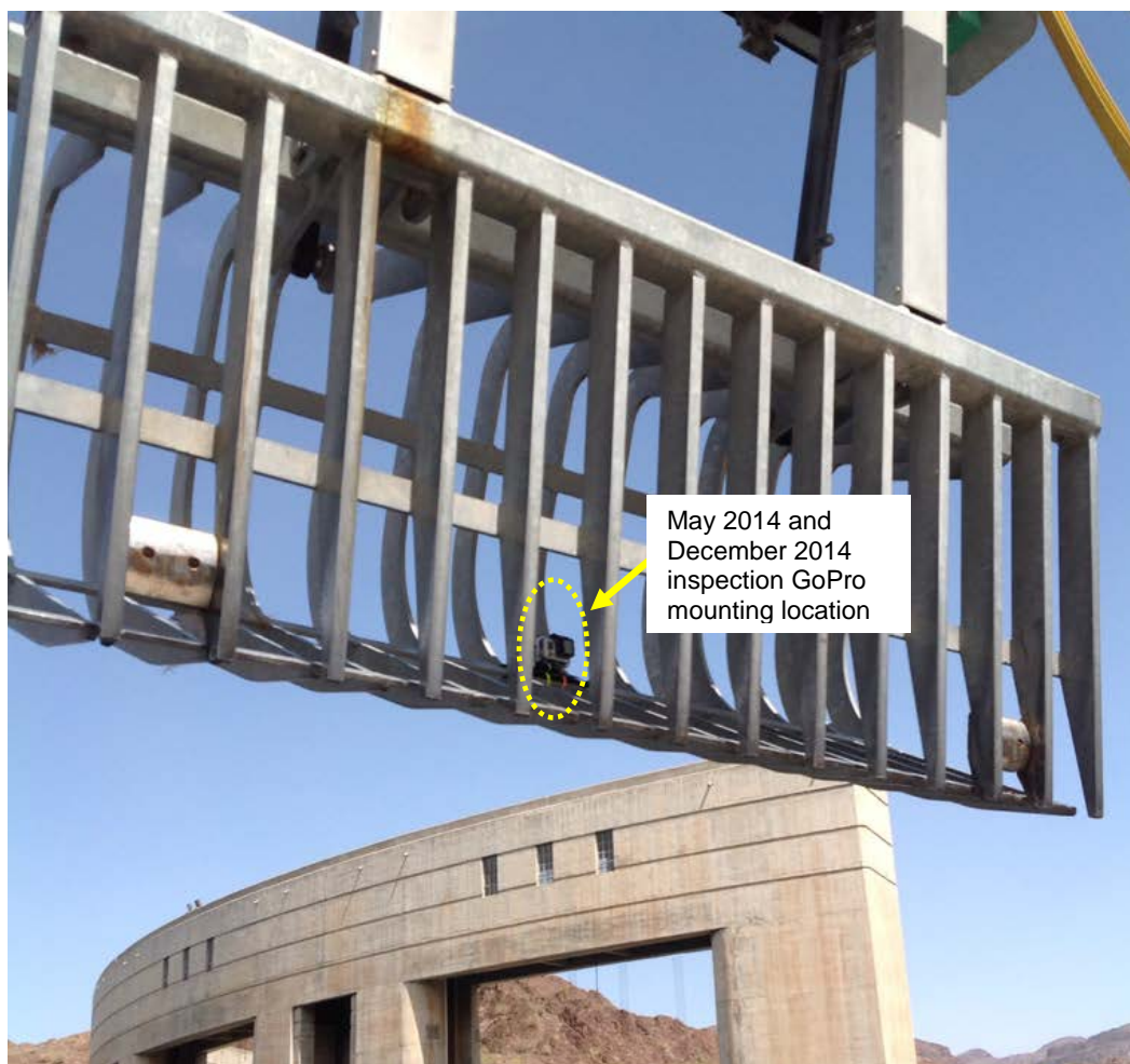
Figure 11.—Trashrack cleaner with GoPro camera mounted.
