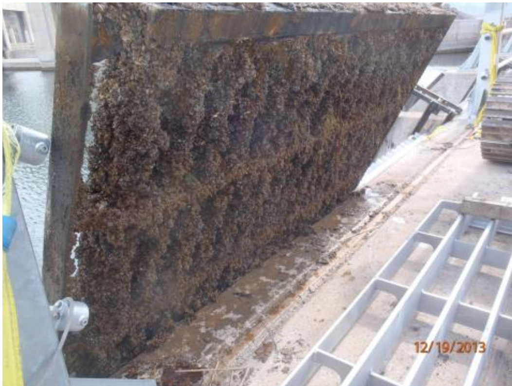
Figure 1.—Existing trashrack heavily fouled with quagga mussels.
