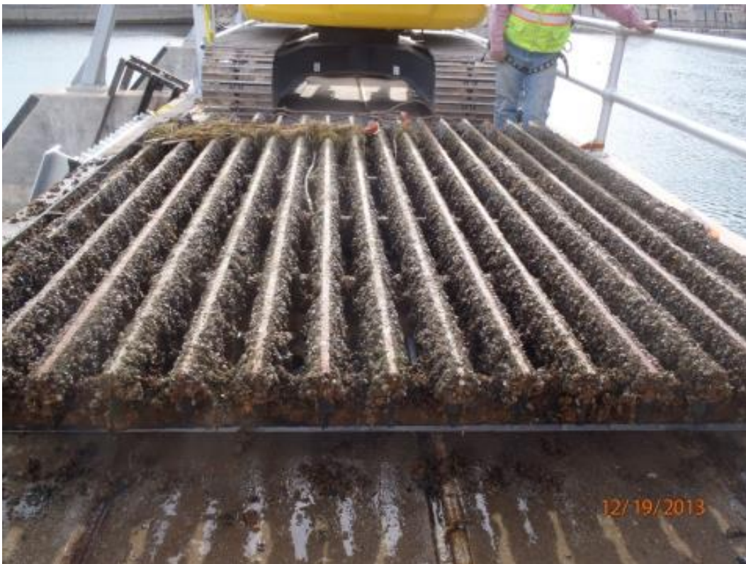
Figure 3.—Existing trashrack, view looking south on trashrack structure.
