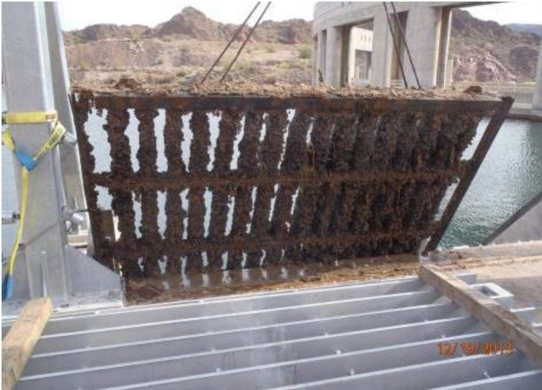
Figure 2.—Existing trashrack, view looking east.
