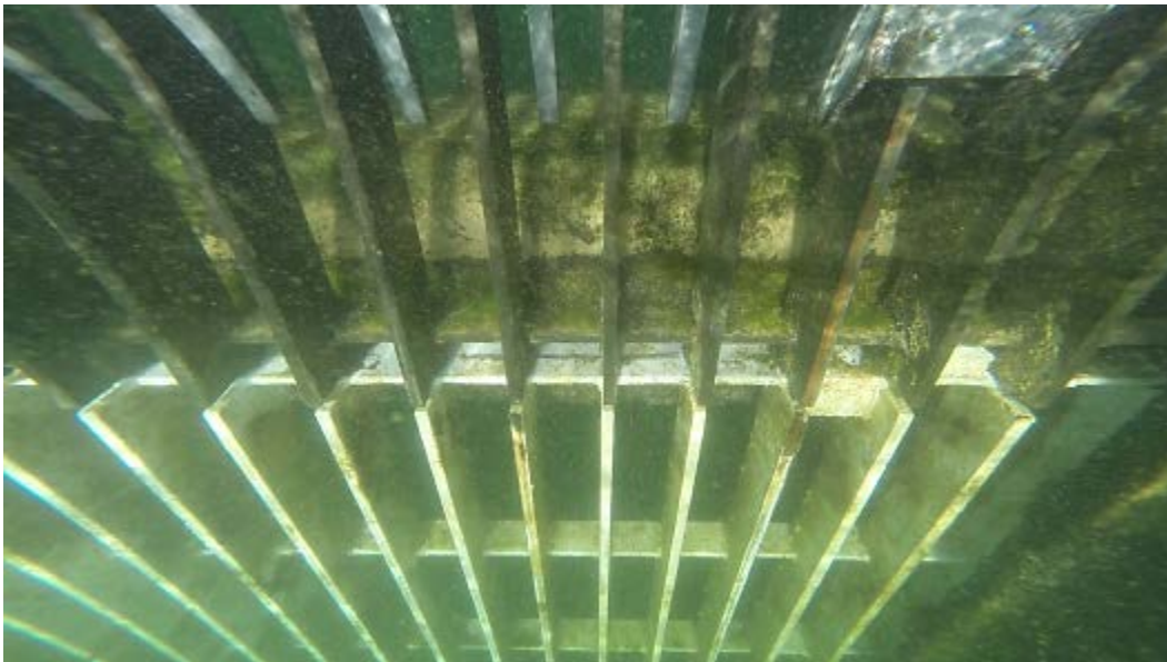
Figure 13.—New galvanized trashrack panel shows corrosion on leading edge where trash rake guide scrapes the surface (third bar from right).
