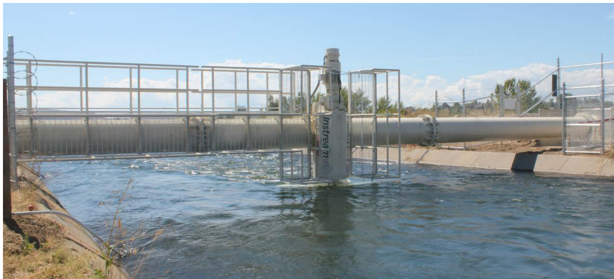
Figure 8 Instream's vertical axis HK turbine operating in the canal (looking downstream).
