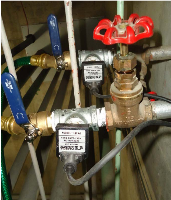
Figure 12 Pressure transducers installed on the Winter-Kennedy taps to measure flow through the hydropower unit at the power plant.
