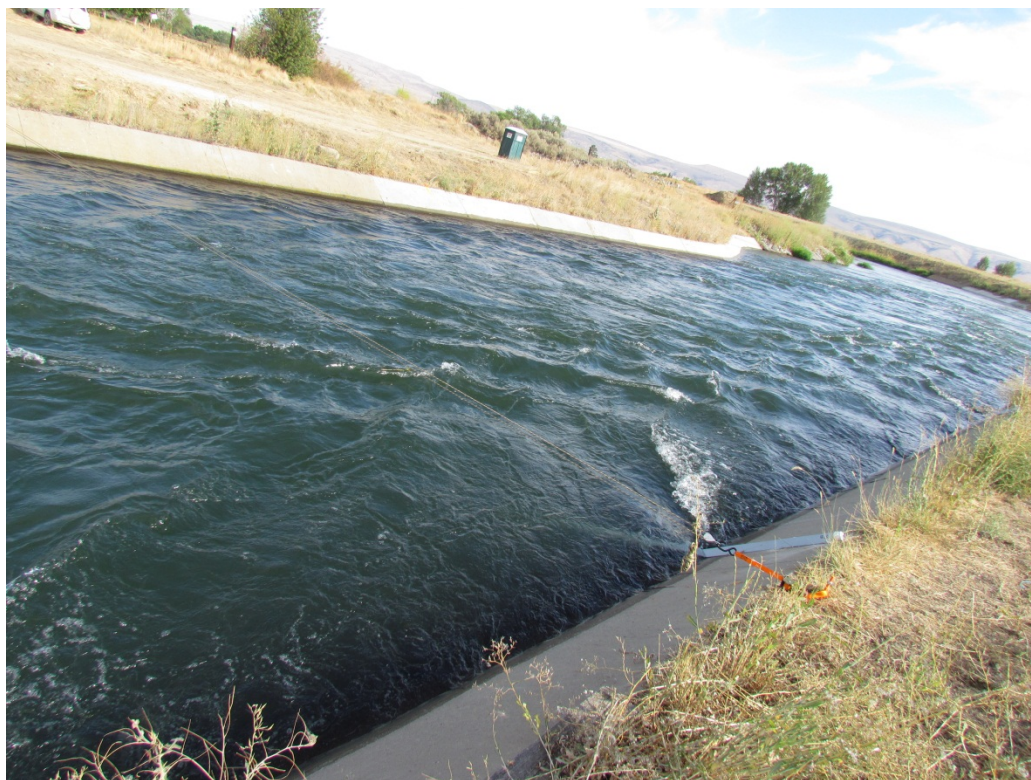
Figure 10 Rough water surface downstream of HK turbine during operation (looking downstream). Flow is entering a transition from lined canal to a wider unlined section.
