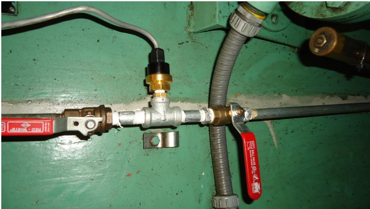
Figure 14 Pressure transducer installed to measure penstock pressure.
