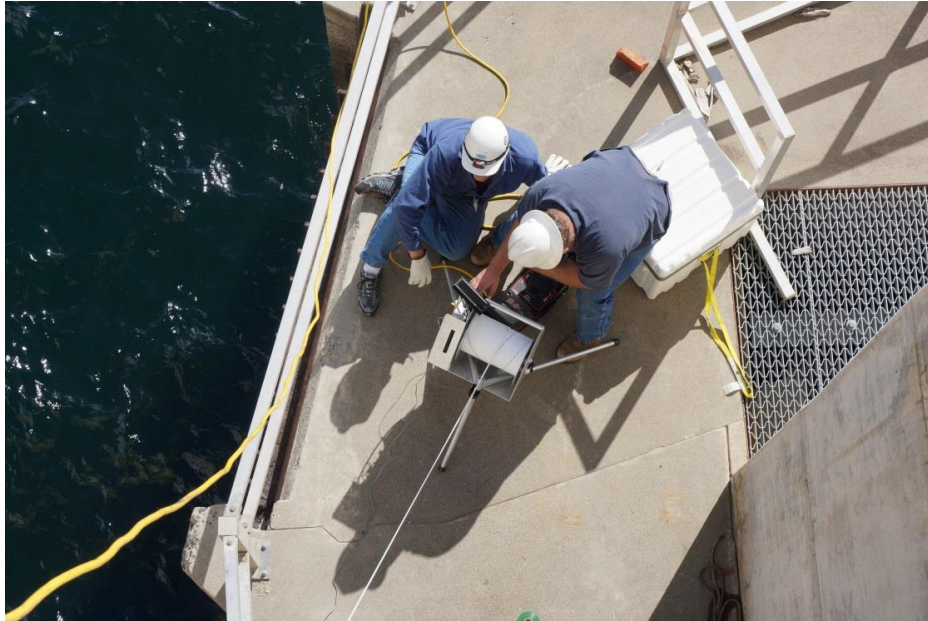
Photo 8.—Grand Coulee personnel monitoring waterstop placement with a well camera.
