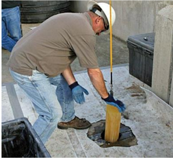
Photo 1.—A section of cylindrical Cylutions waterstop being placed into a core hole.
