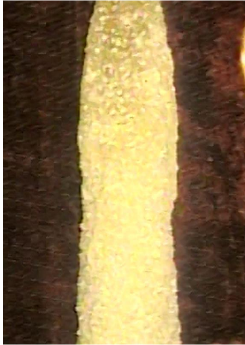
Photo 10.—Waterstop material creating a mound on the face of the joint.
